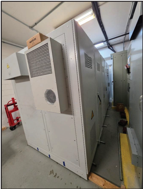
Figures 7 & 8: Voltage Regulation Transformer placed in ATS room awaiting final positioning
