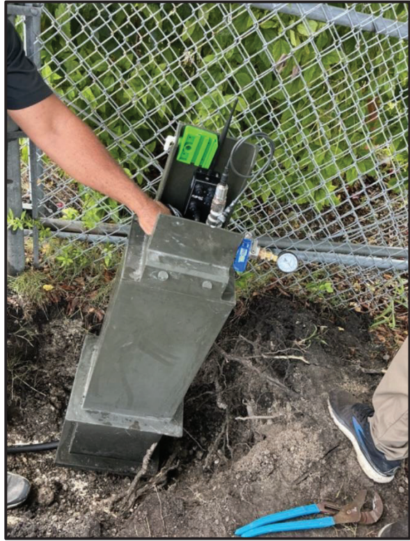
Figures 5 & 6: Installation of Pressure Monitoring
