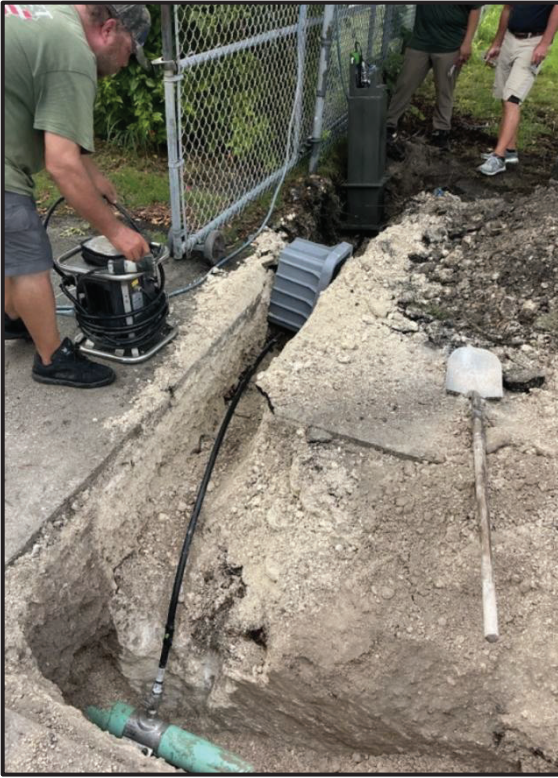
Figures 5 & 6: Installation of Pressure Monitoring
