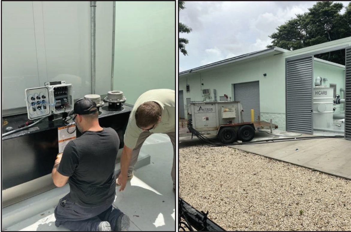
Figures 9 & 10: Vacuum Station A Load Testing & Start-up
