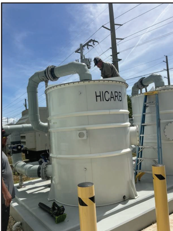
Figures 1 & 2: Additional Maintenance Flanges Installed at Vacuum Stations I and JK.
