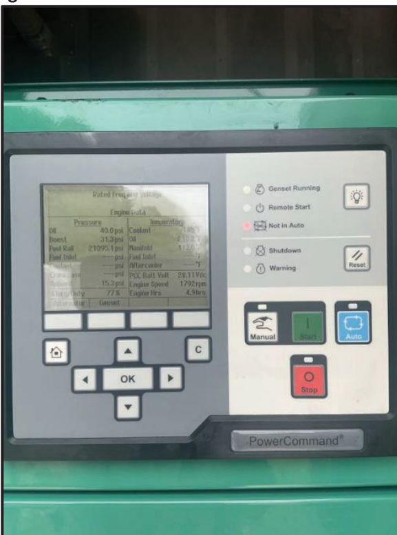
Figures 3 & 4: Vacuum Station D Final Wiring & 100% Load Testing Parameters
