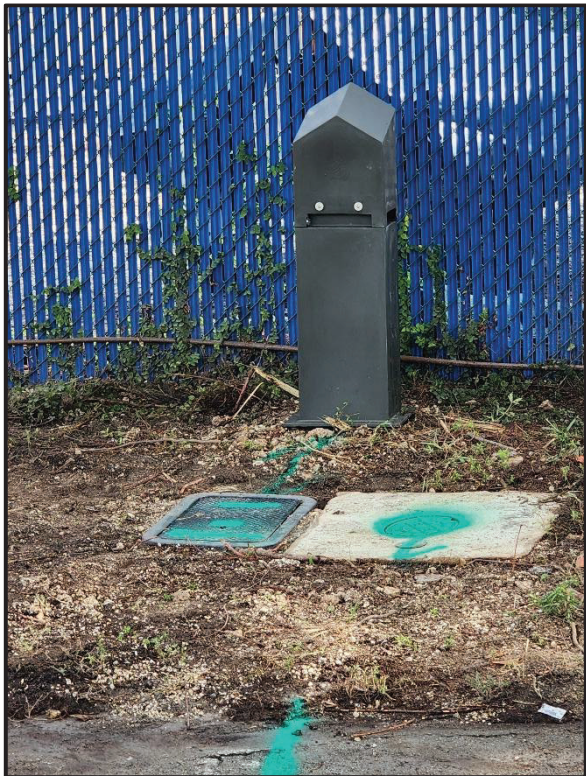
Figures 3 & 4: Installed FM Monitoring Sensor and Site Restoration
