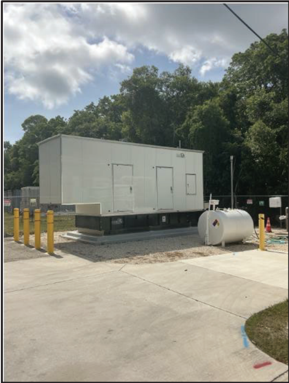
Figures 1 & 2: Generators Fastened in Place at Stations A and D.
