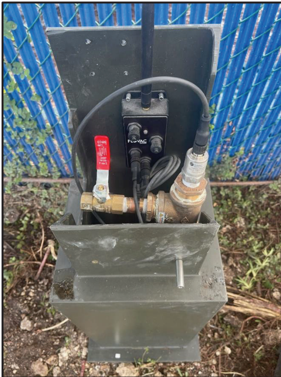
Figures 3 & 4: Installed FM Monitoring Sensor and Site Restoration
