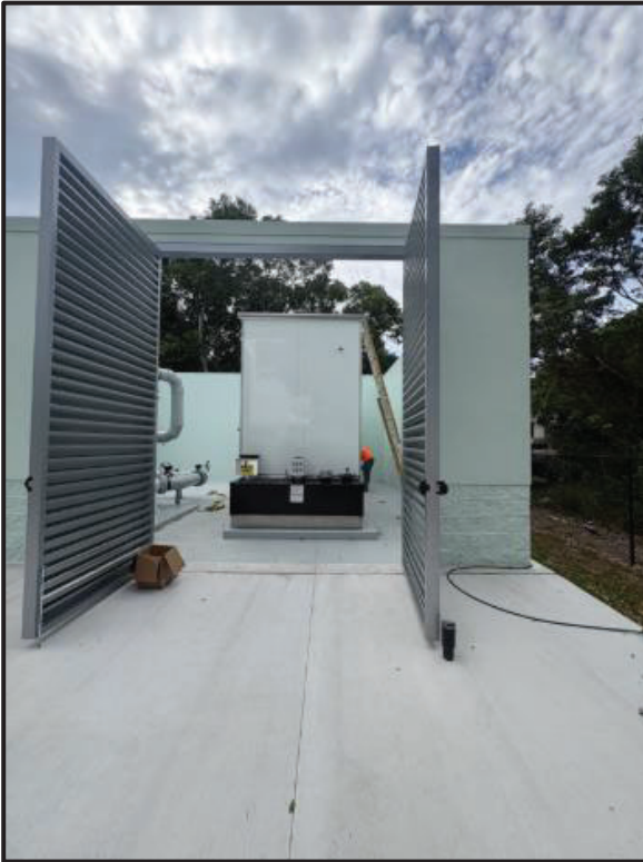
Figures 1 & 2: Generators Fastened in Place at Stations A and D.
