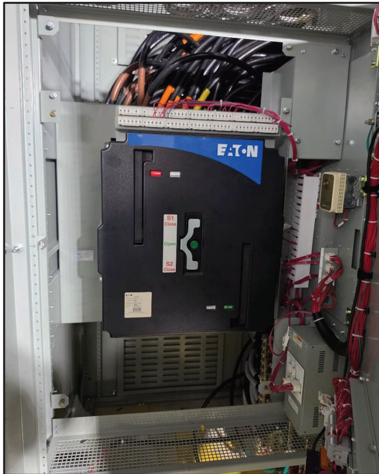
Figures 2 & 3: Finalized Conductor Connections in New 2500 kVA ATS Project Construction Photos Cont.
