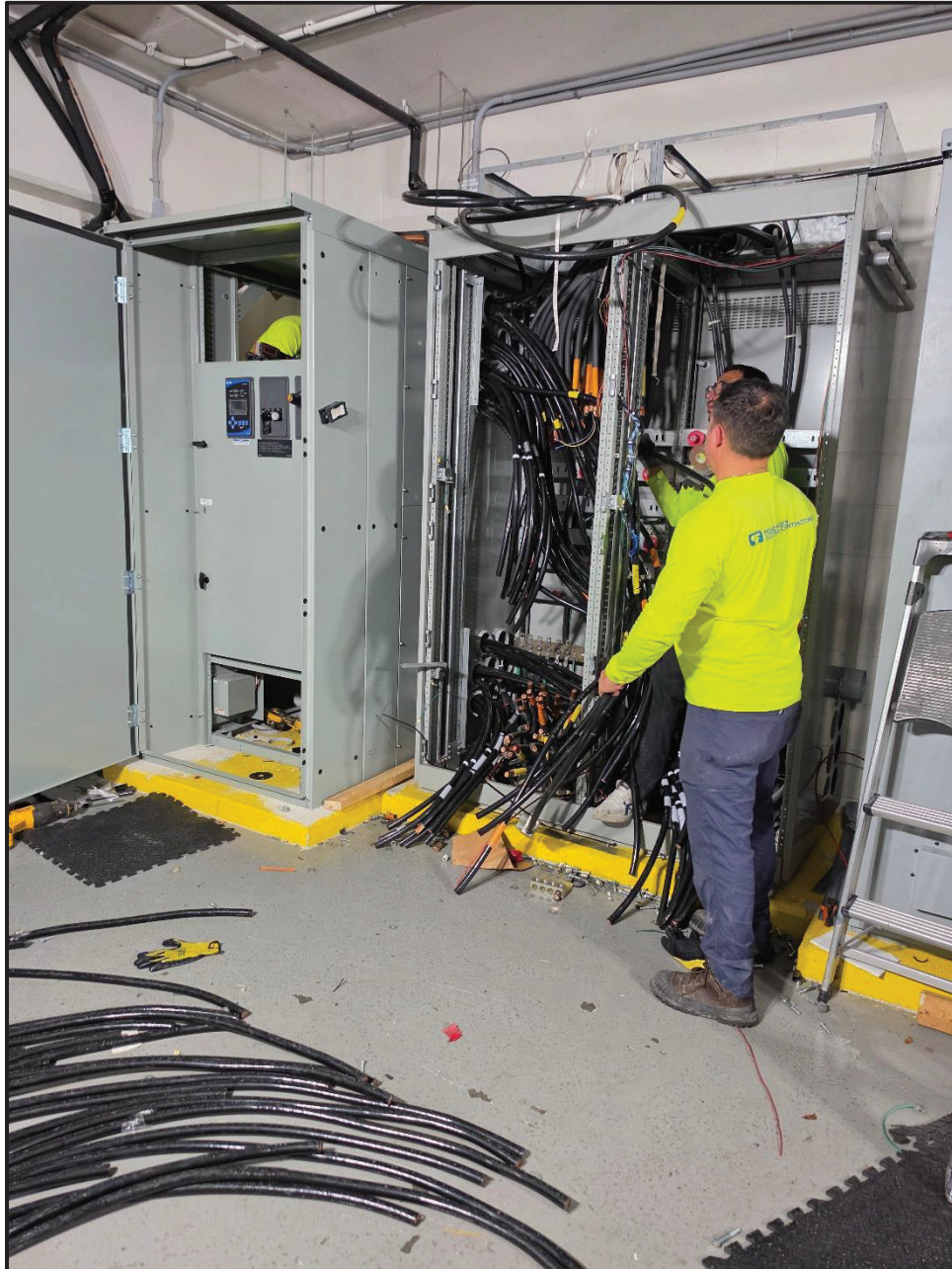
Figure 1: Pedro Falcon Connecting Main Service Conductors to New 2500 kVA ATS
