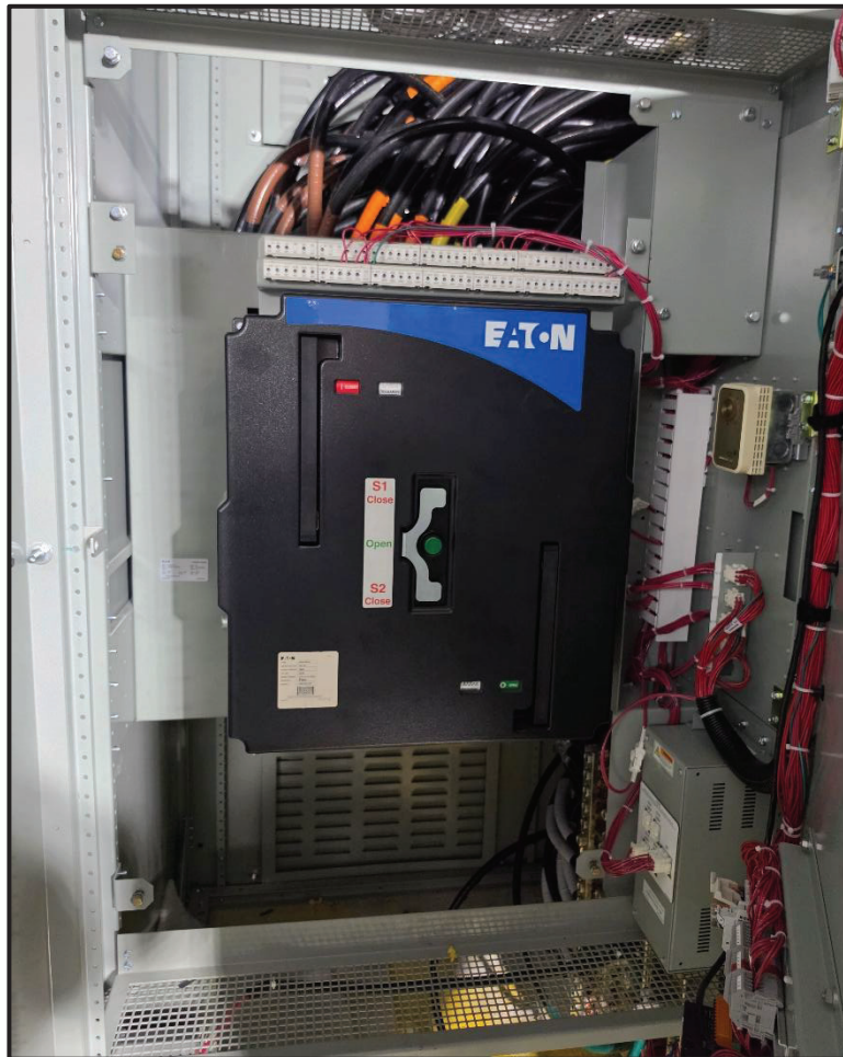
Figures 2 & 3: Finalized Conductor Connections in New 2500 kVA ATS Project Construction Photos Cont.
