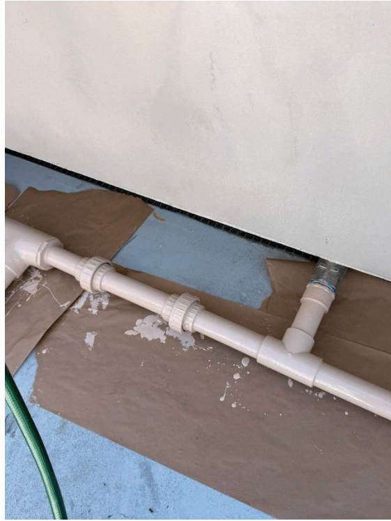
Figures 5 & 6: New Drain lines for Evoqua Filter Installed, Tested and Painted by Reynolds
