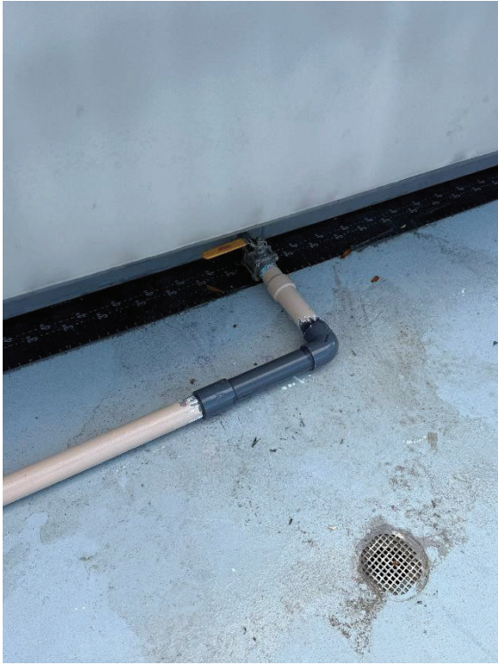
Figures 5 & 6: New Drain lines for Evoqua Filter Installed, Tested and Painted by Reynolds
