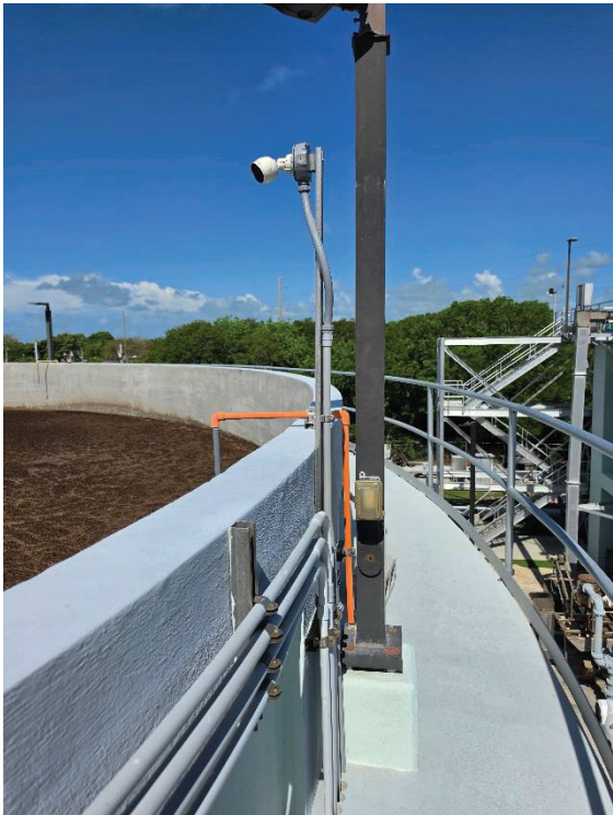
Figures 3 & 4: New Cameras and Conduit installed on all Tanks and Equipment Pads
