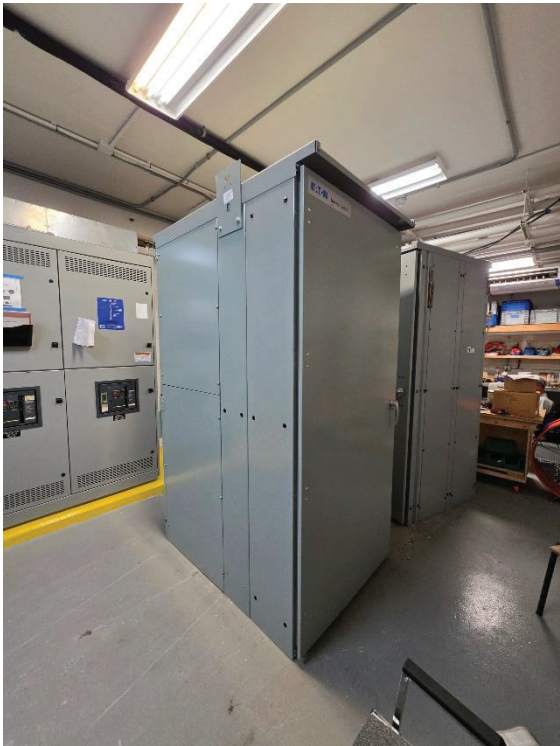
Figures 5 & 6: New 2500A ATS Delivered and Placed on Painted Equipment Pad
