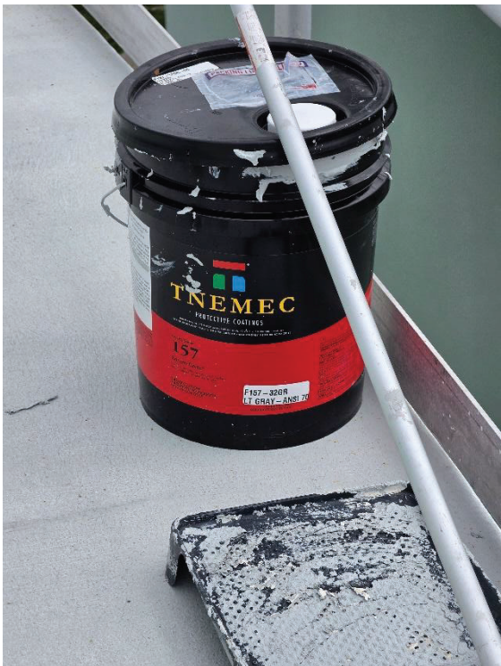
Figures 3 & 4: Pedro Falcon Using Tnemec Series 157 Top Coating on the SBR and Building Walkways
