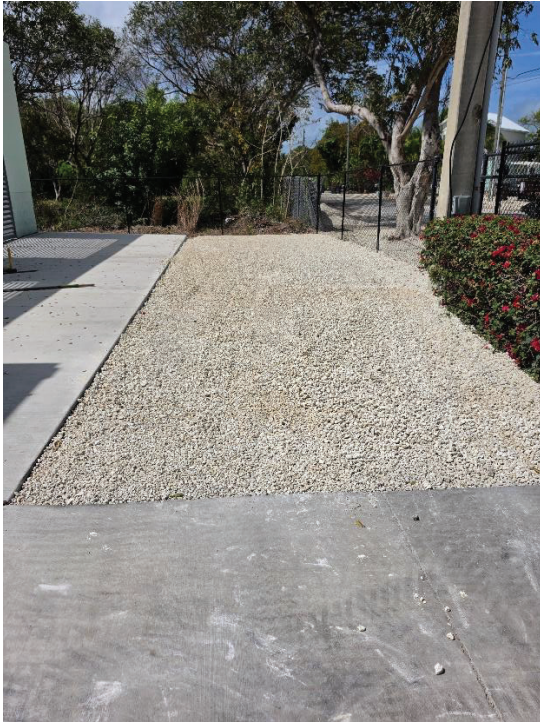
Figure 9 & 10: Site Restoration & #57 Stone Installed at Vacuum Station A & E
