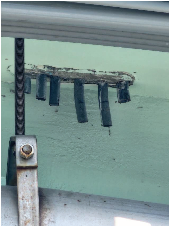
Figures 5 & 6: Pedro Falcon Workers Cutting Old Conduit Flush and Filling Them with Epoxy Cement
