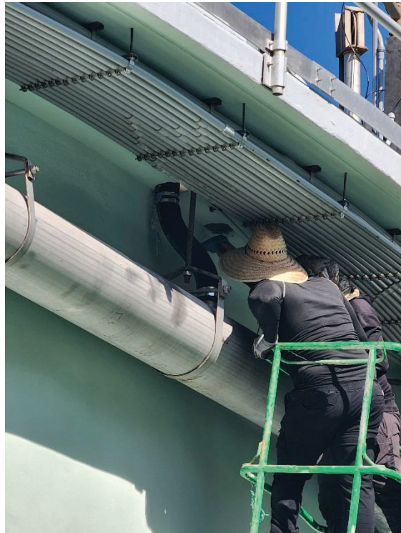
Figures 5 & 6: Pedro Falcon Workers Cutting Old Conduit Flush and Filling Them with Epoxy Cement
