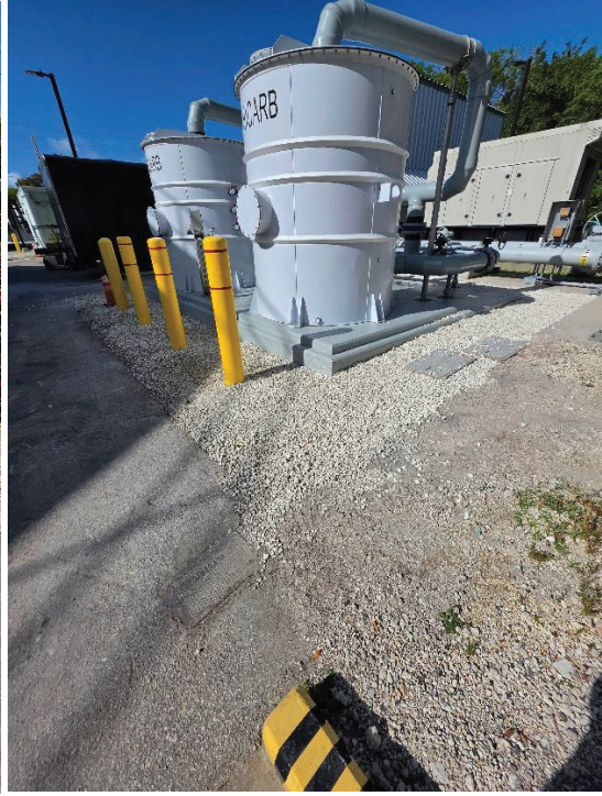
Figure 9 & 10: Site Restoration & #57 Stone Installed at Vacuum Station A & E
