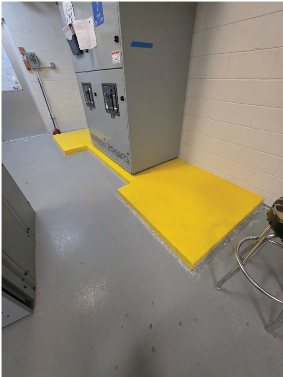
Figures 3 & 4: Concrete Equipment Pad for ATS and Disconnect Painted
