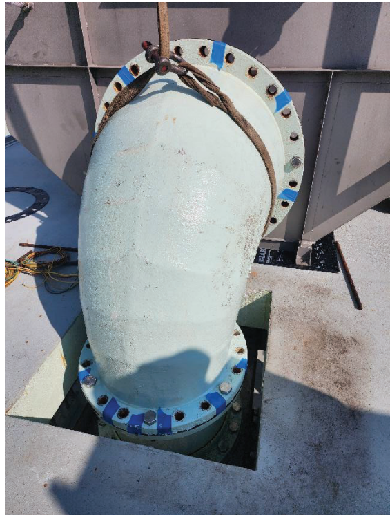
Figures 7 & 8: Disk Filter Fitting with Existing Piping Network
