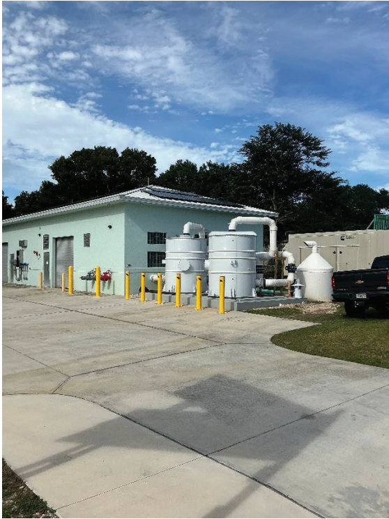
Figure 9 & 10. Bollards Installed At Vacuum Stations E & I
