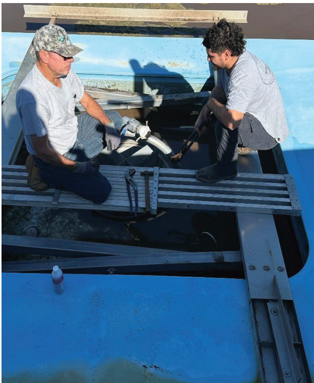
Figures 5 and 6: SBR decanter ballast hose replacement
