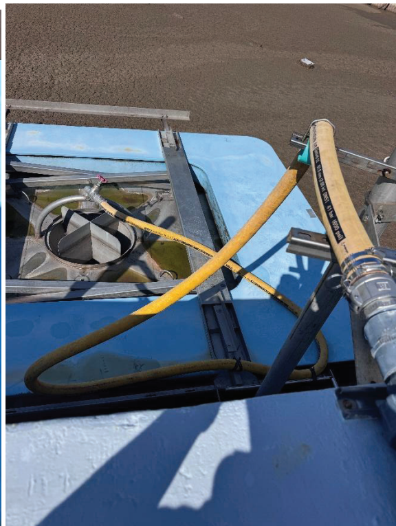
Figures 5 and 6: SBR decanter ballast hose replacement
