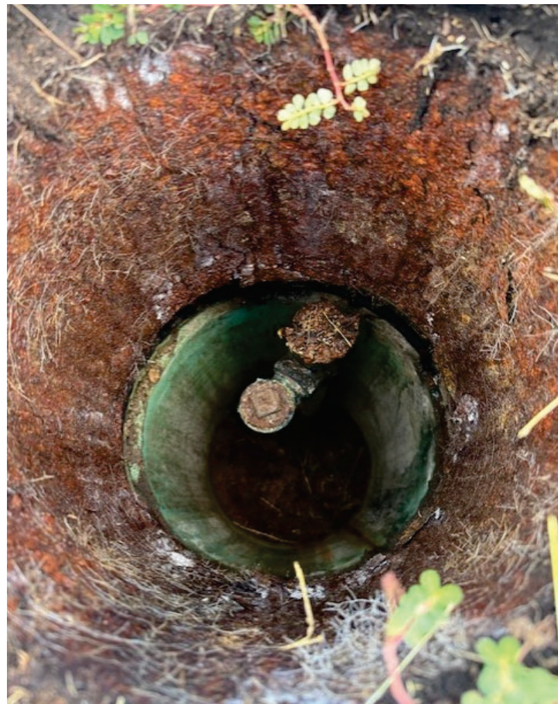
Corrosion of an existing 2" Blow Off Tap
