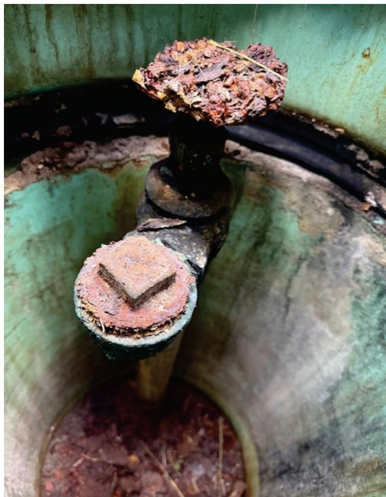
Corrosion of an existing 2" Blow Off Tap
