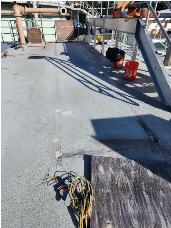
Figures 7 & 8. Reynolds On-Site Repairing The Damage To The Coating On The Filter Platform
