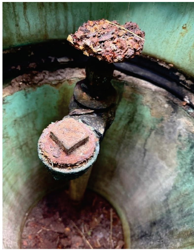
Corrosion of an existing 2" Blow Off Tap
