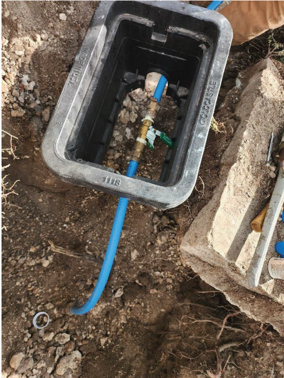
Figures 1 & 2. Installation Of The First Force Main Pressure Monitoring Equipment For The Collection System Monitoring Project
