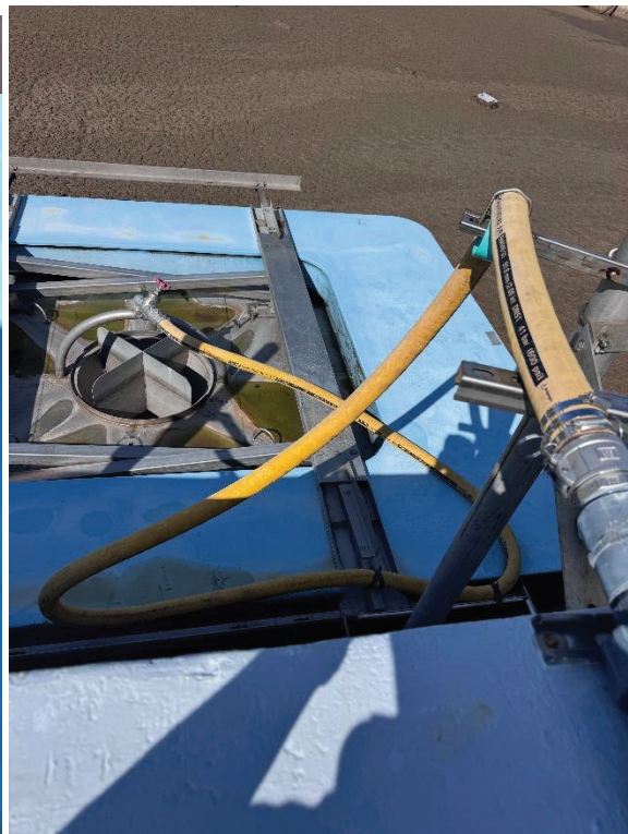
Figures 5 and 6: SBR decanter ballast hose replacement
