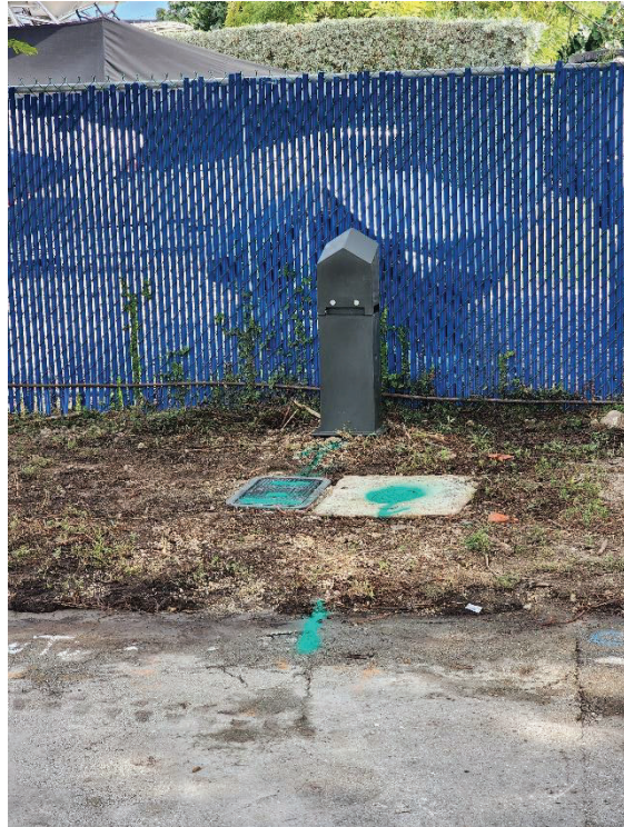
Figures 1 & 2. Installation Of The First Force Main Pressure Monitoring Equipment For The Collection System Monitoring Project
