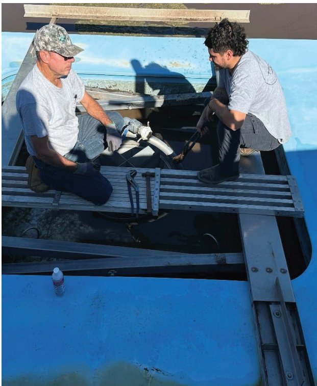
Figures 5 and 6: SBR decanter ballast hose replacement
