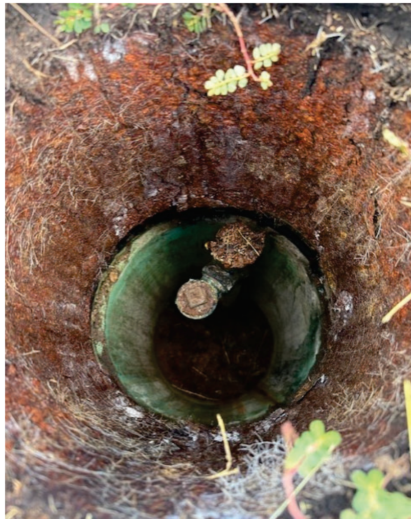
Corrosion of an existing 2" Blow Off Tap
