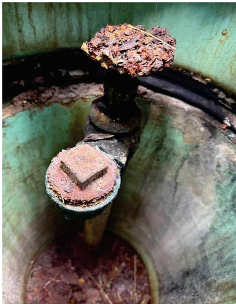
Corrosion of an existing 2" Blow Off Tap
