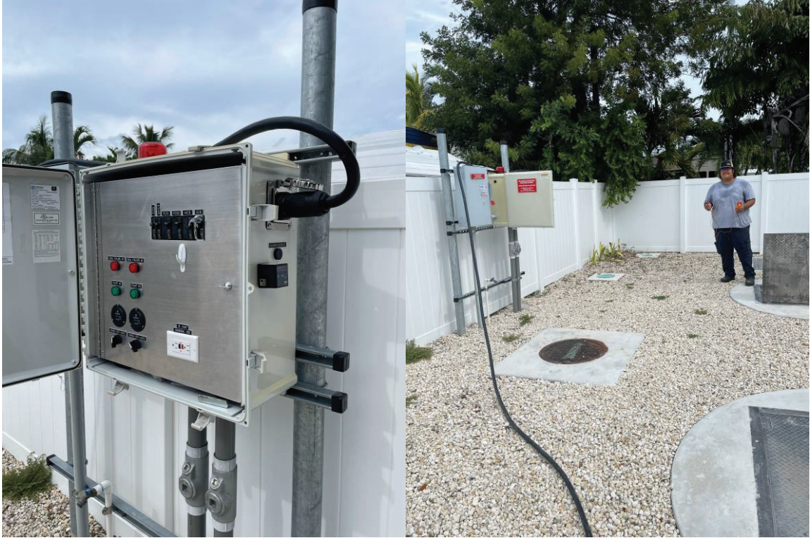
Figures 1 and 2: Generator cable connected to lift station control panel
