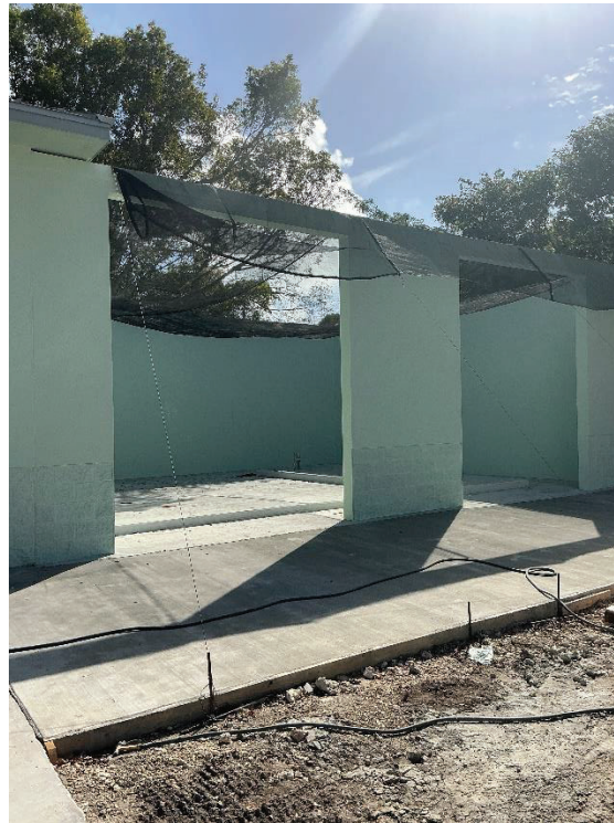
Figure 11. Concrete Driveway Installed And Final Coating Applied On Vacuum Station A Building Extension.
