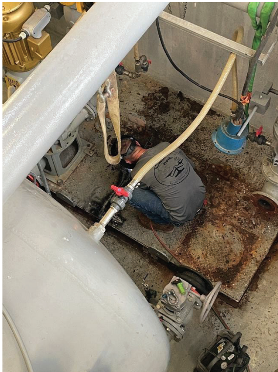
Figure 2: Pump removed and steel skid cutting
