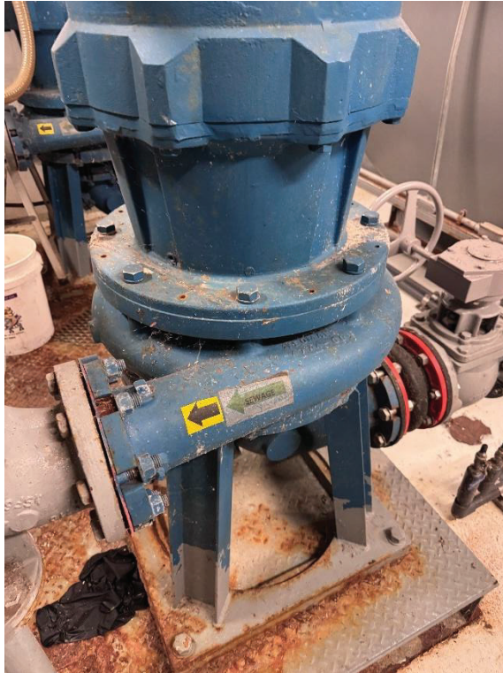
Figure 1: Old pump and rusted pump skid
