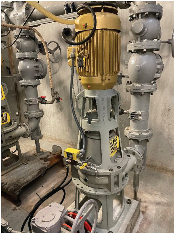
Figures 8 and 9: New pump installed, wired and seal water system plumbed.
