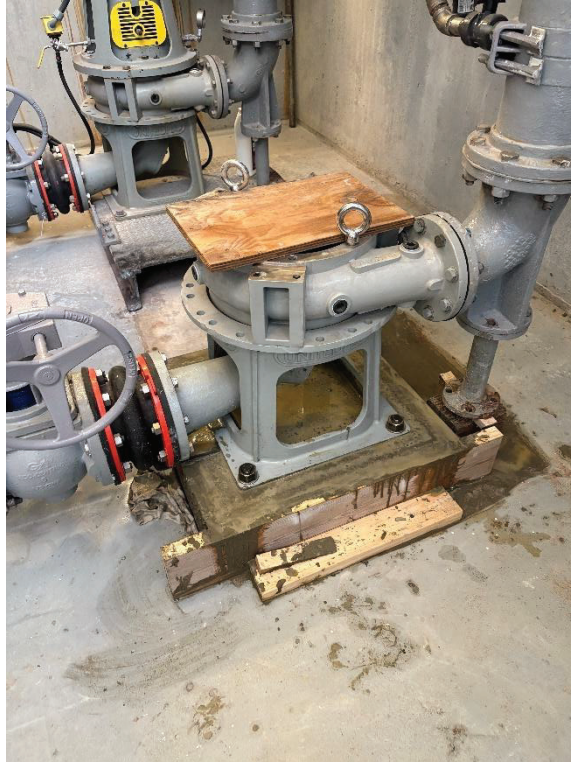
Figure 7: Grout pump base formed and poured
