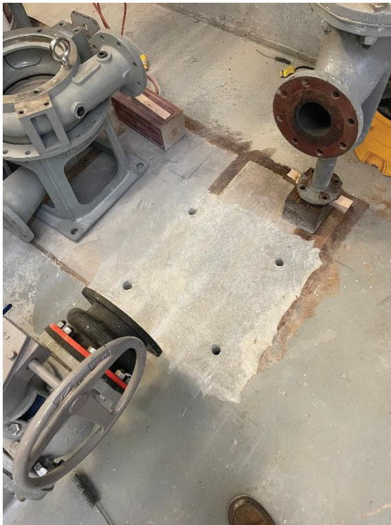
Figures 5 and 6: Grout base prep work
