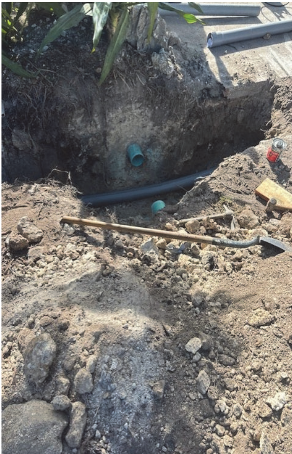
Picture 3: Damaged Section Removed
