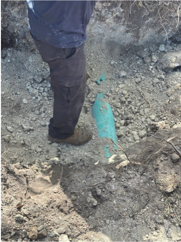
Picture 3: Damaged Section Removed
