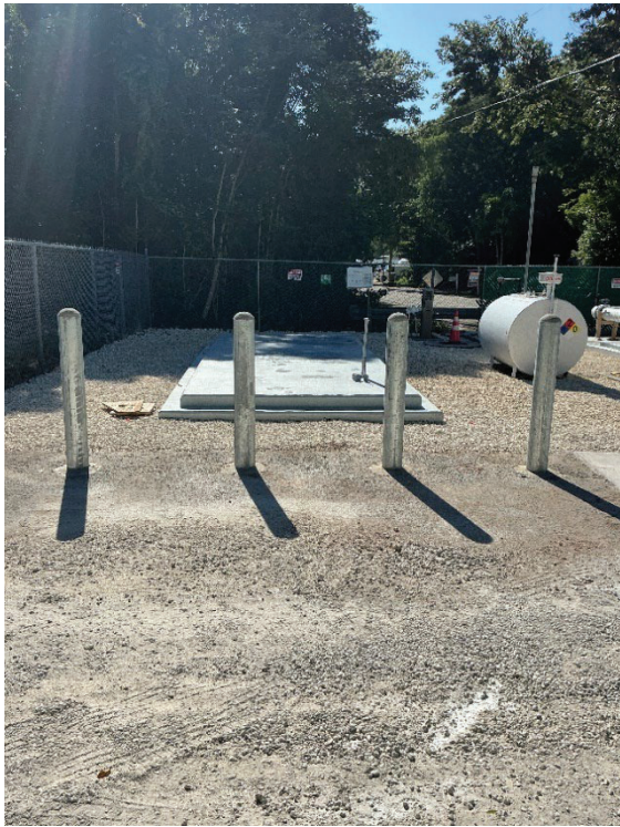
Figure 9 & 10. #57 Stone and Bollards installed at Vacuum Station D.
