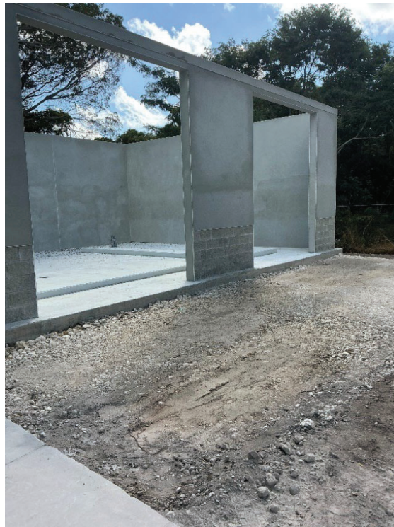
Figure 11. Stucco applied on Vacuum Station A Building Extension.
