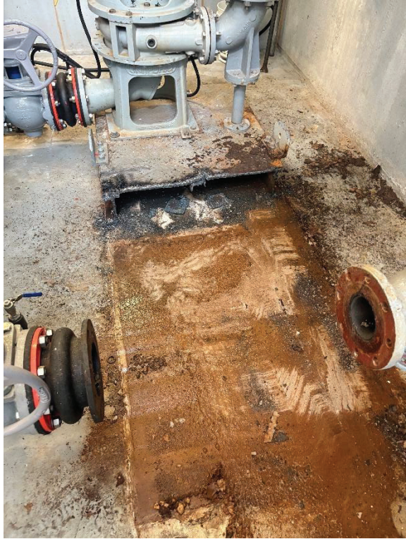
Figures 3 and 4: Steel skid removal
