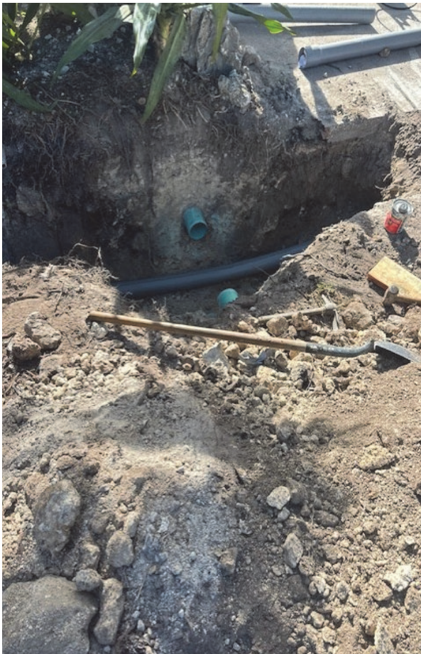
Picture 3: Damaged Section Removed
