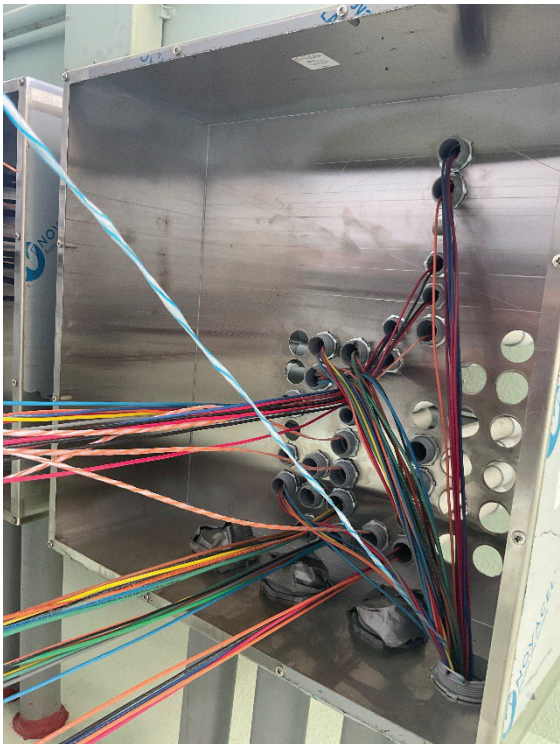
Figures 3 & 4. Routing Wire through a Junction Box into Panels For Equipment For Final Connection
