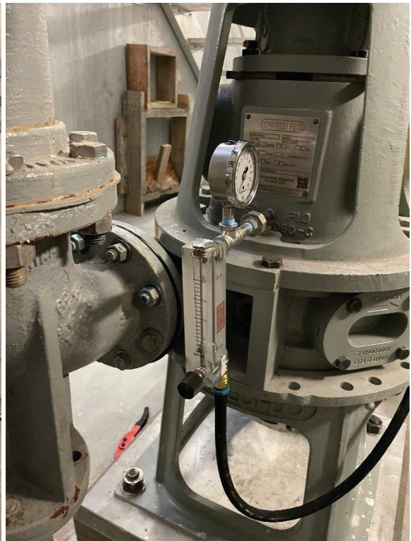
Figures 8 and 9: New pump installed, wired and seal water system plumbed.
