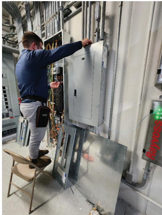
Figures 3 & 4. Routing Wire through a Junction Box into Panels For Equipment For Final Connection
