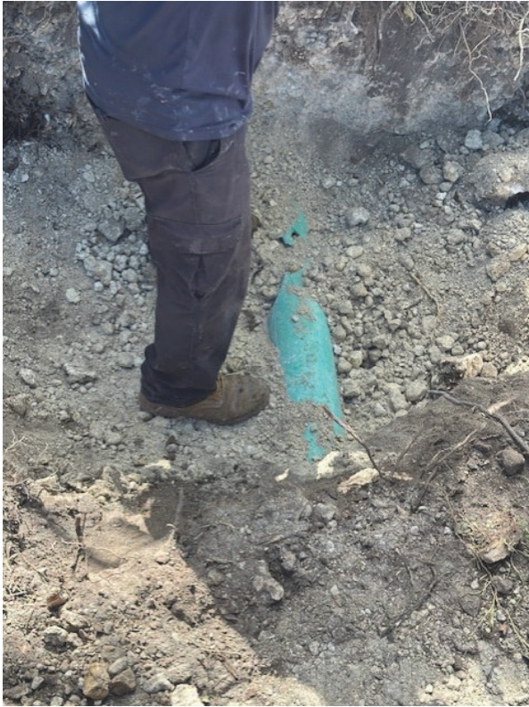
Picture 3: Damaged Section Removed
