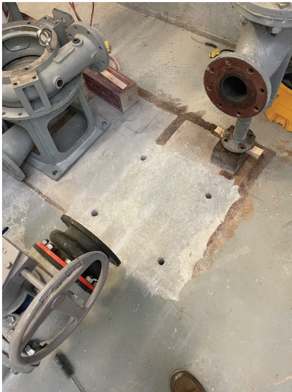
Figures 5 and 6: Grout base prep work
