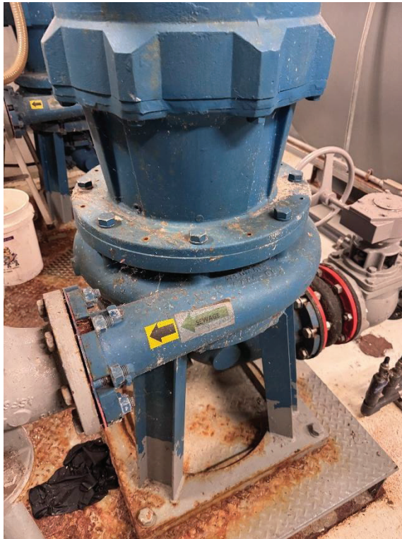
Figure 1: Old pump and rusted pump skid
