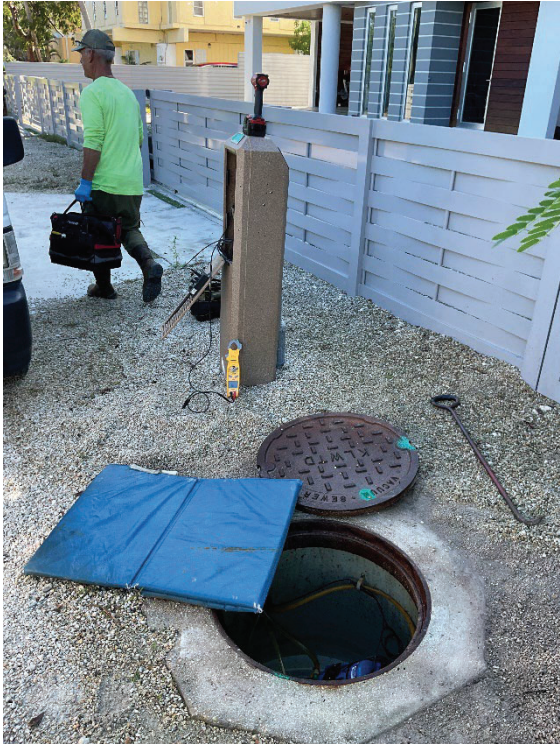
Figures 1 & 2. Y-Cable cleaned and reassembled in Basin B For The Collection System Monitoring Project
