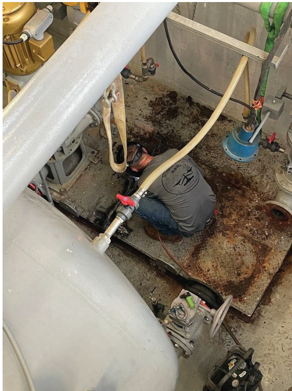
Figure 2: Pump removed and steel skid cutting
