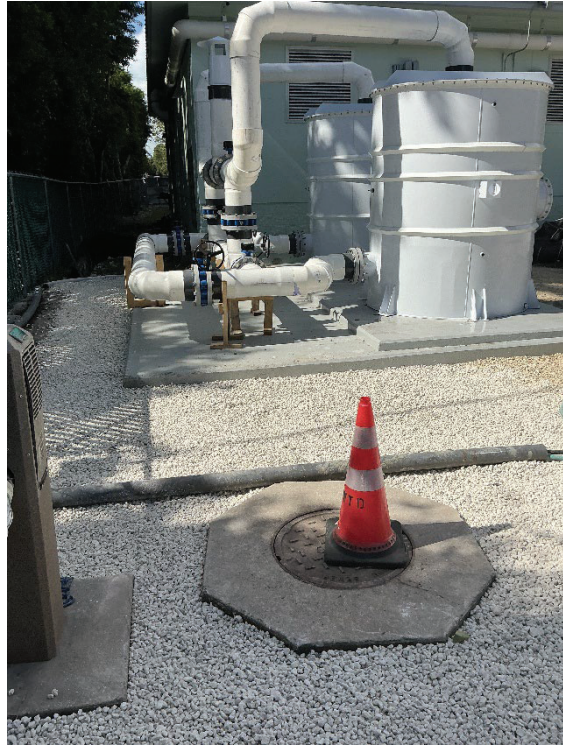
Figure 9 & 10. #57 Stone and Bollards installed at Vacuum Station D.
