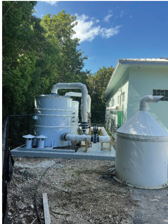
Figure 9 & 10. Odor Control System Piping Nearly Completed.
