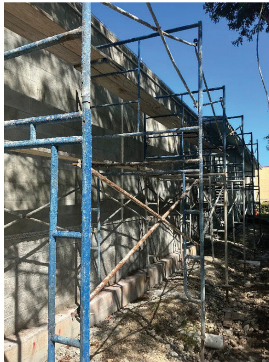
Figure 11. Scaffolding Installed To Begin Finish Work At Vac Station A
