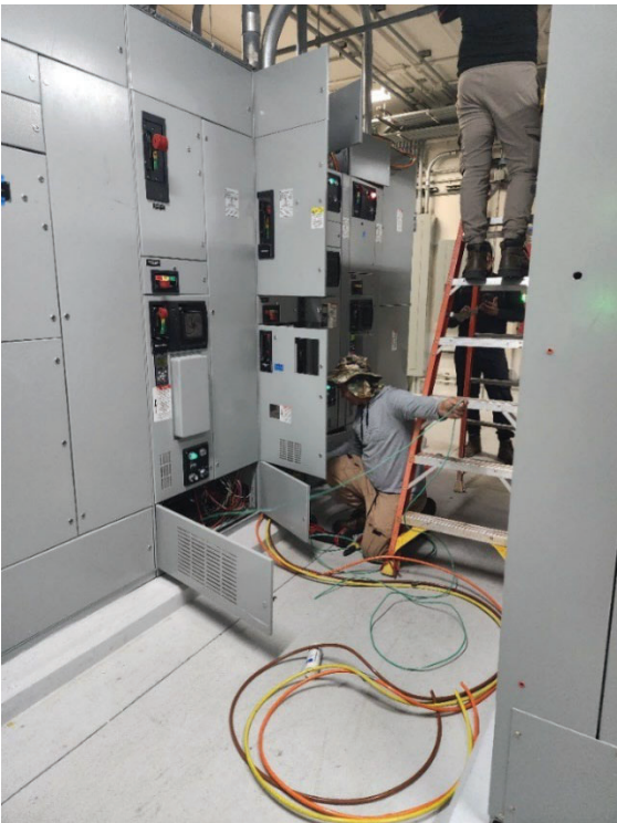
Figures 3 & 4. Routing Wire Into MCC For Equipment Preparing For Shutdown For Final Connection
