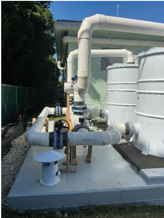
Figure 9 & 10. Odor Control System Piping Nearly Completed.
