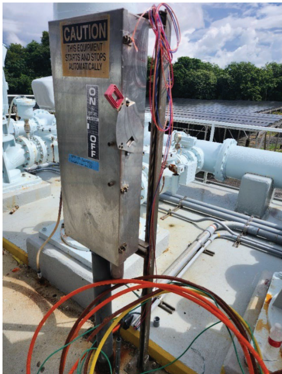
Figures 5 & 6. Wire Pulled Through New Conduit At The Injection Well Pumps
