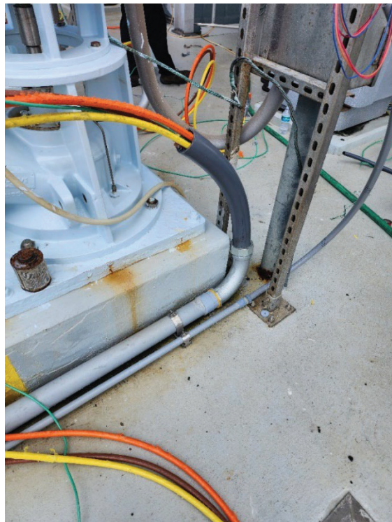
Figures 5 & 6. Wire Pulled Through New Conduit At The Injection Well Pumps
