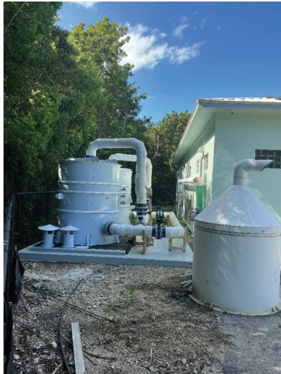
Figure 9 & 10. Odor Control System Piping Nearly Completed.
