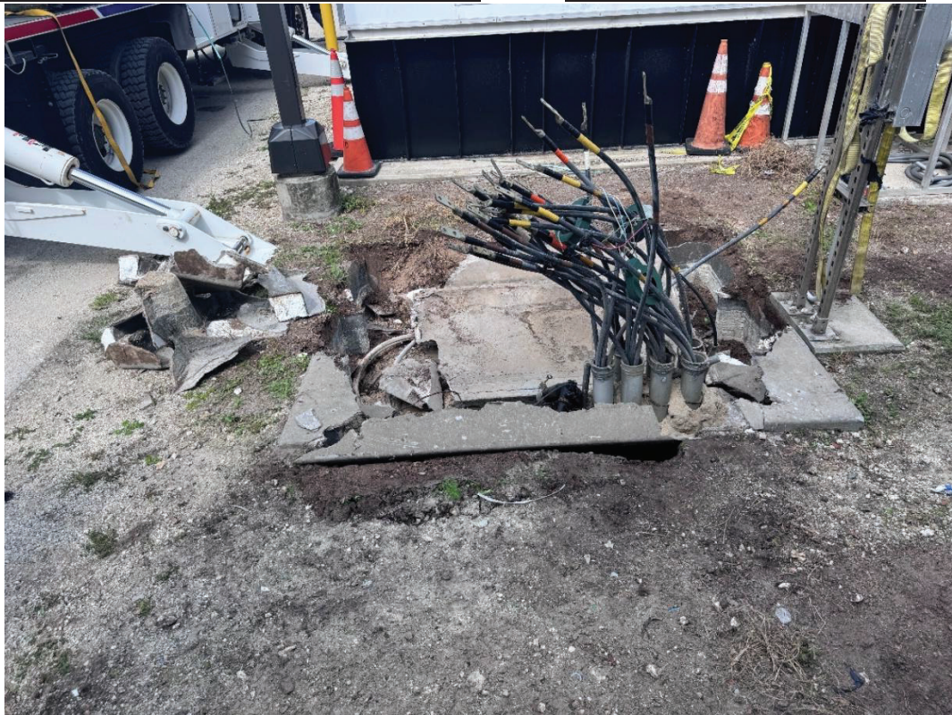
Figure 9: Old pad demolition
