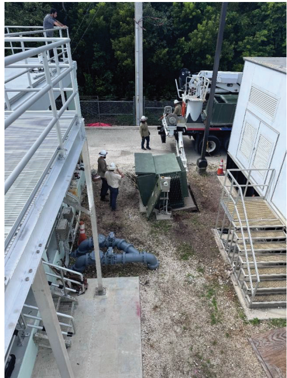
Figure 8: Transformer removal
