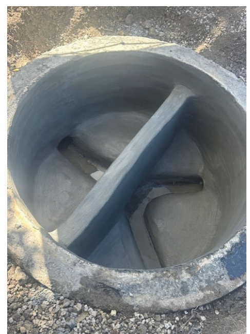
Finished Product 1' Geopolymer Liner
