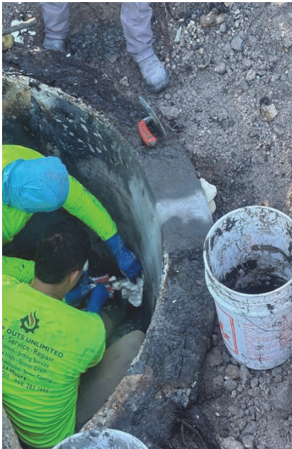
Applying Infiltration Control Chemical Grouting
