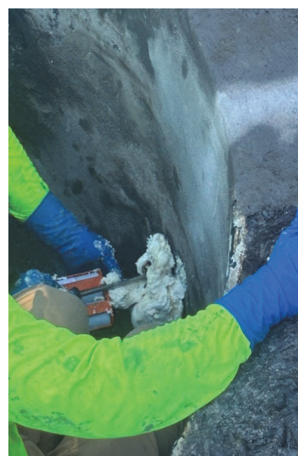
Applying Infiltration Control Chemical Grouting
