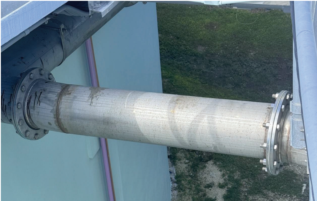
Figure 6: New flange gaskets installed
