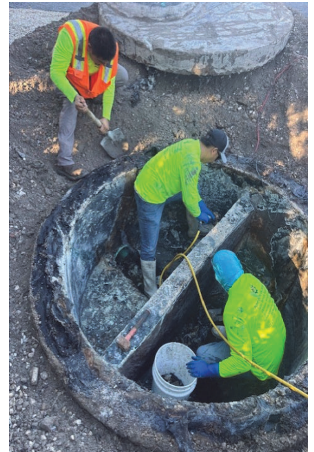
Finished Product 1' Geopolymer Liner
