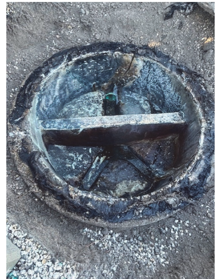
Removal of Existing Epoxy
