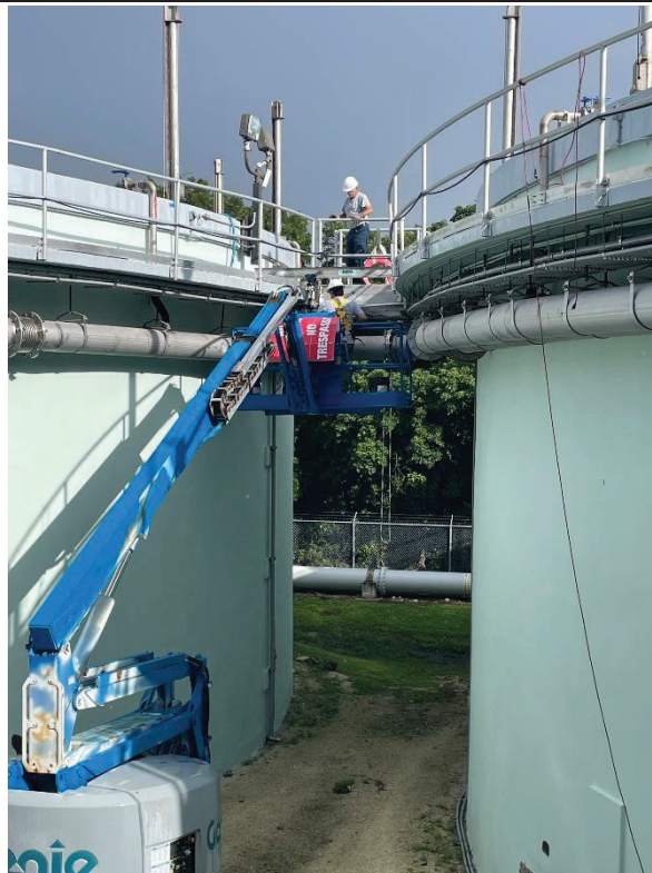
Figure 4: Facilities technicians preparing the work area
