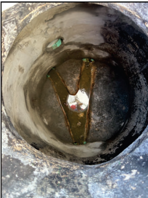
Infiltration Control - Chemical Grouting
