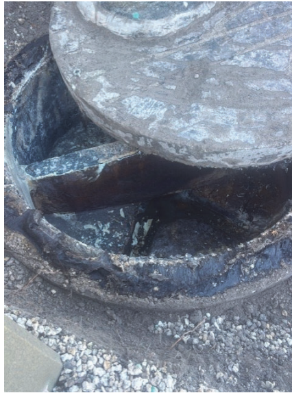
Removal of Existing Epoxy
