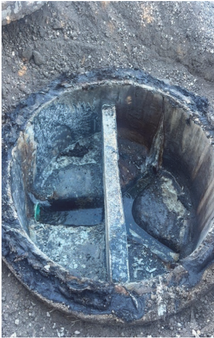
Applying Infiltration Control Chemical Grouting
