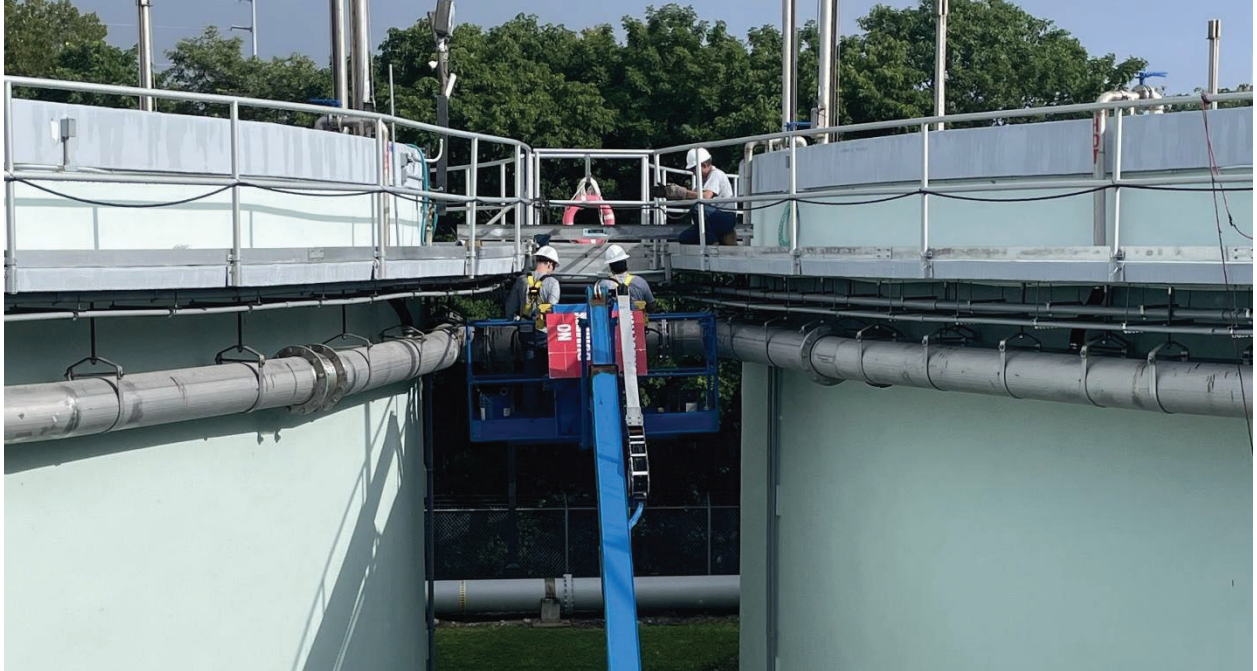
Figure 5: Facilities technicians preparing temporary airline supports
