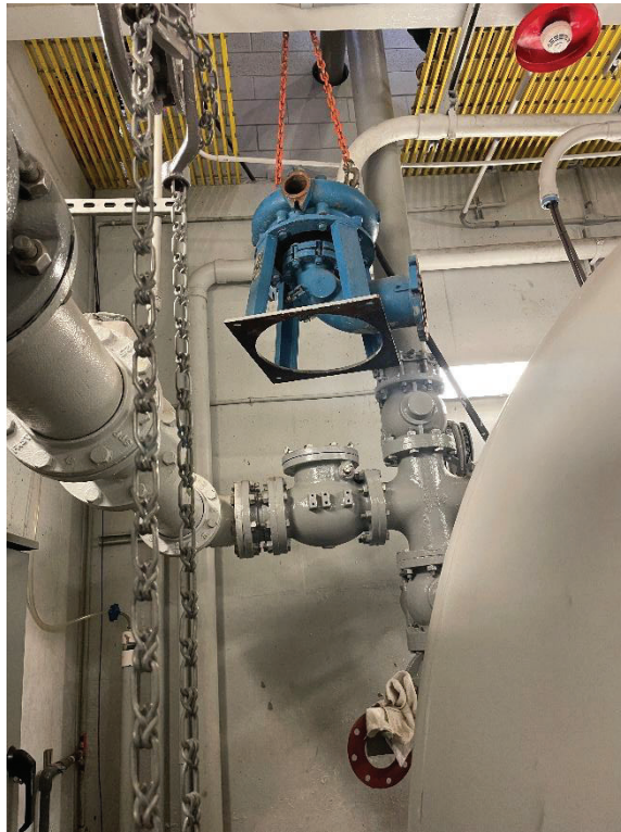
Figure 11: Spare sewage pump volute and pump base being lowered into tank vault
