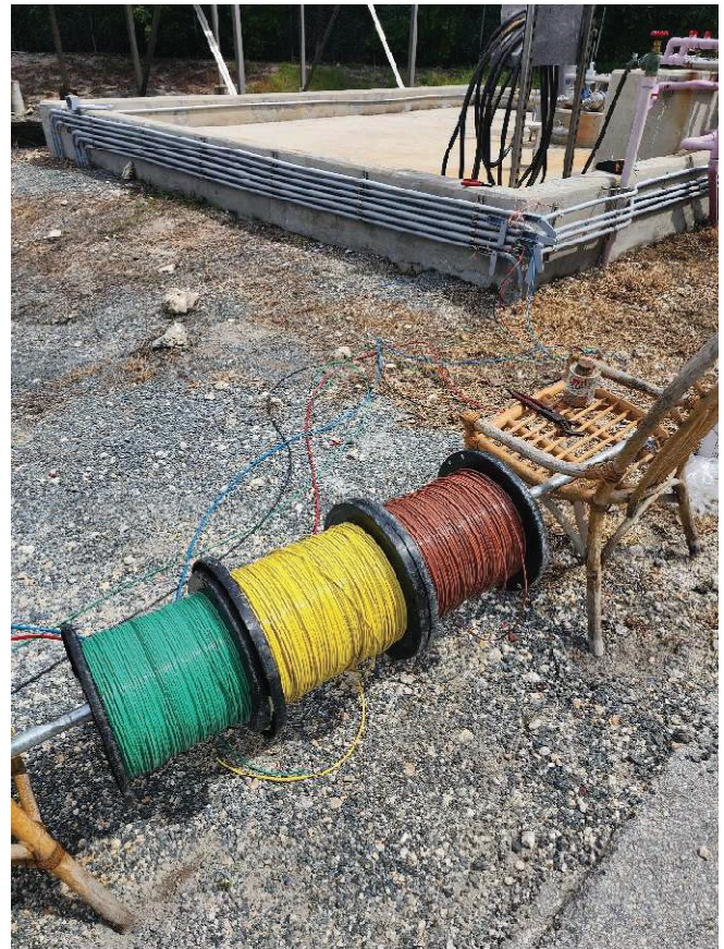
Figures 5 & 6. Wire for pulling through conduit and wires actively pulled through conduit
