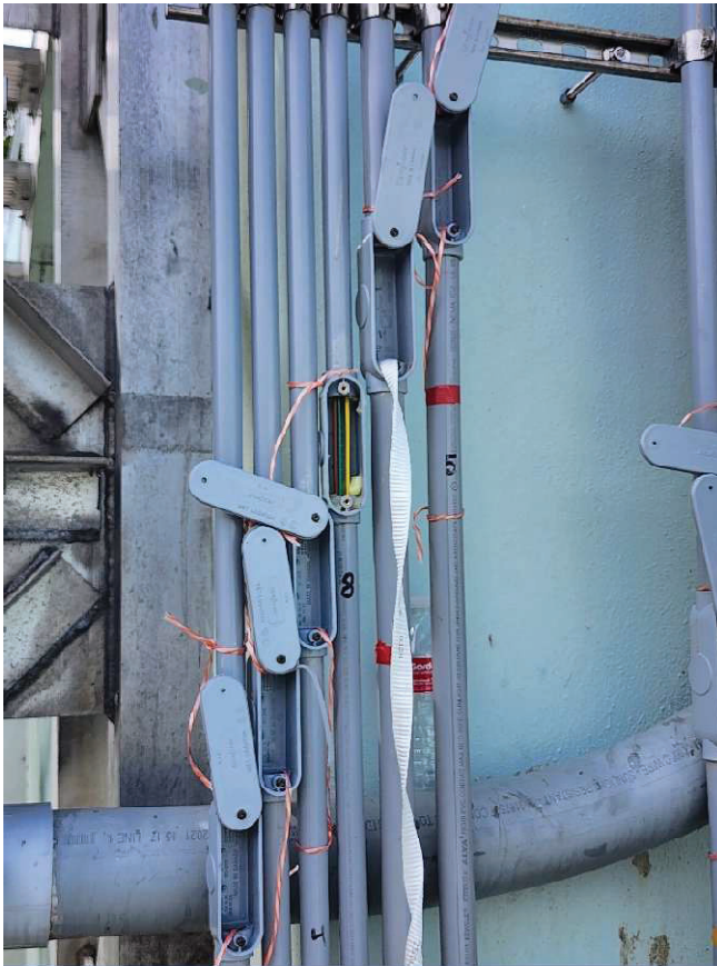
Figures 5 & 6. Wire for pulling through conduit and wires actively pulled through conduit
