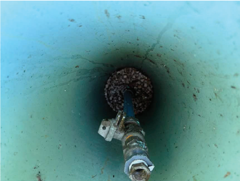
Figures 1 & 2. Existing Force Main Tap to be Used for Pressure Monitoring
