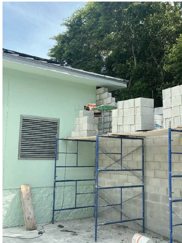
Figure 8. Construction of New CMU Wall Extension and Foundation at Vac Station A
