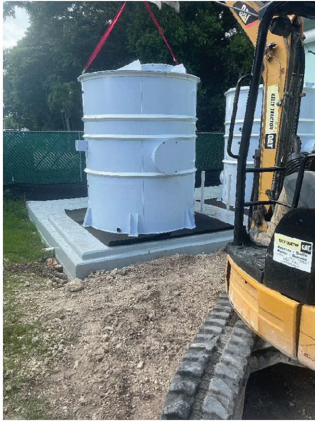
Figure 7. Odor Control Tanks delivered
