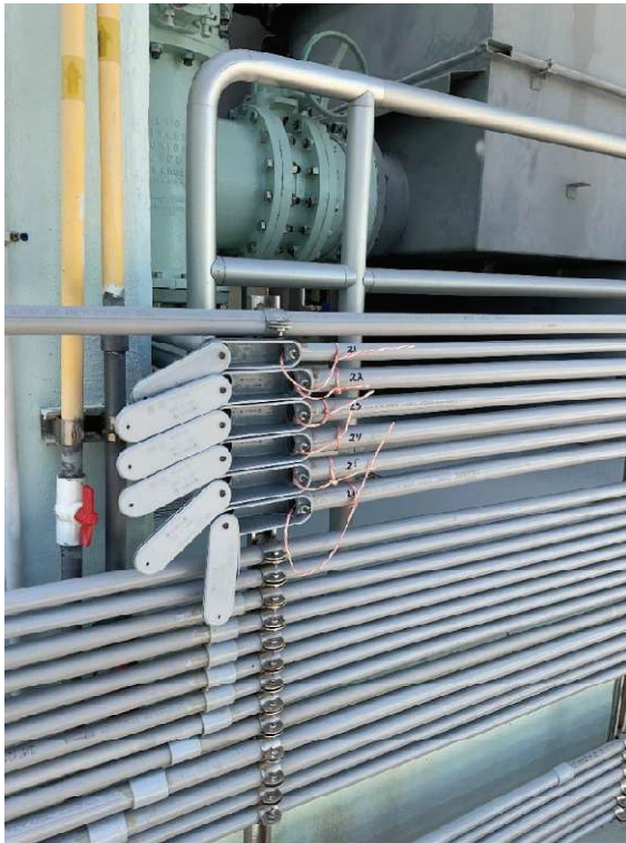
Figures 3 & 4. Pull Strings in Conduits Along the East Side of the Disinfection Basin
