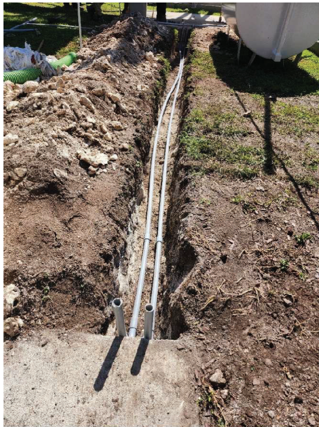
Figures 5 & 6. PVC Conduits Installed Between KLWTD & Islamorada Salinity Probe & Flow Meters
