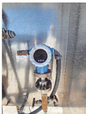
IW-1 Pressure transmitter
