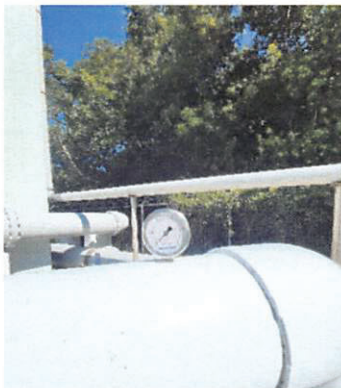
Class V Backup well pressure gauge WACS 100121
