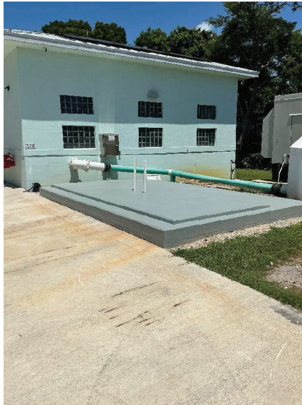
Figure 7. New Odor Control Slab at Vacuum Station I
