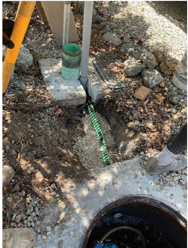
Figures 1 & 2. Collection System Monitoring IVC Concrete Installing Conduit in Trench
