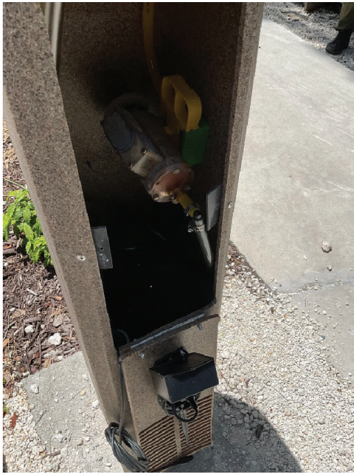
Figures 5 & 6. FloVac Checking Pit is Online After Pulling Hose Lines through Conduit
