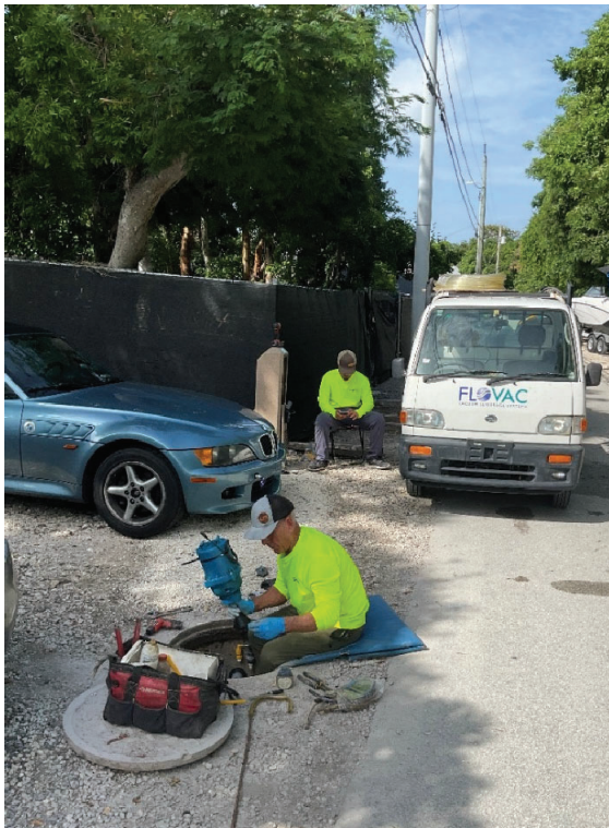
Figures 3 & 4. Collection System Monitoring FloVac Installing Hose Lines and Swapping Valves
