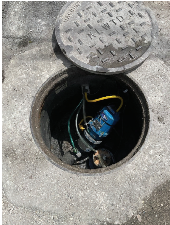
Figures 3 & 4. Collection System Monitoring FloVac Installing Hose Lines and Swapping Valves
