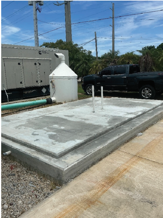
Figures 13 & 14. New Odor Control slabs at Vacuum Stations G and I
