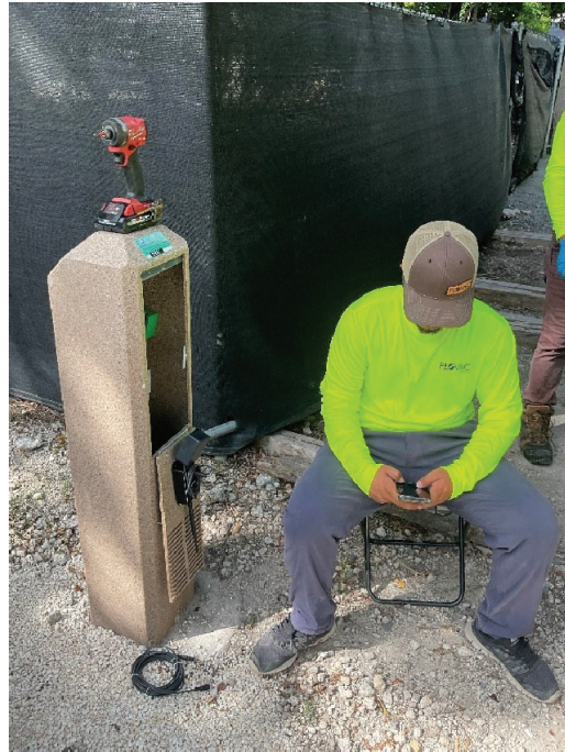
Figures 5 & 6. FloVac Checking Pit is Online After Pulling Hose Lines through Conduit
