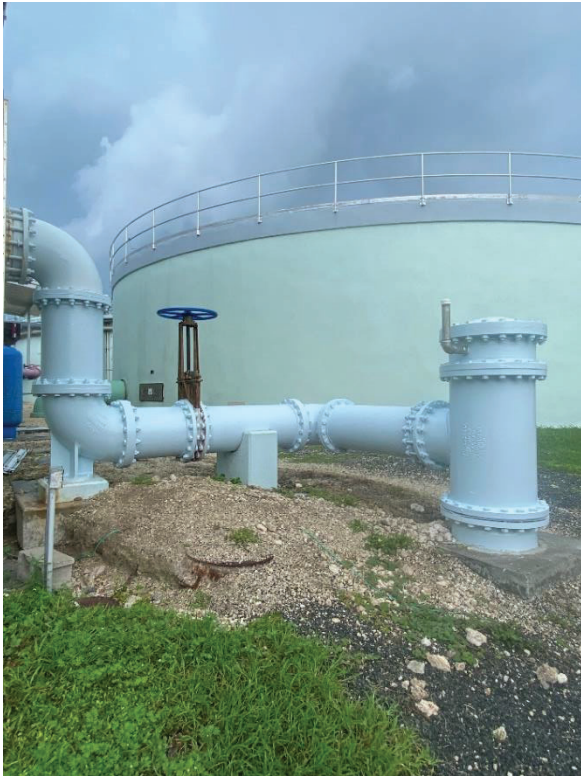
Figures 7 and 8: Well piping treated and painted.
