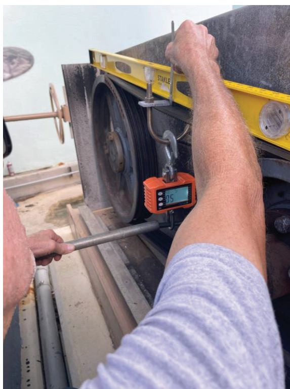
Figure 11: Digester motive pump belt adjustment.
