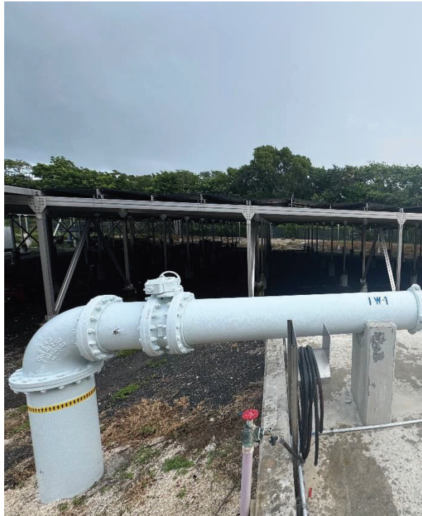
Figures 7 and 8: Well piping treated and painted.
