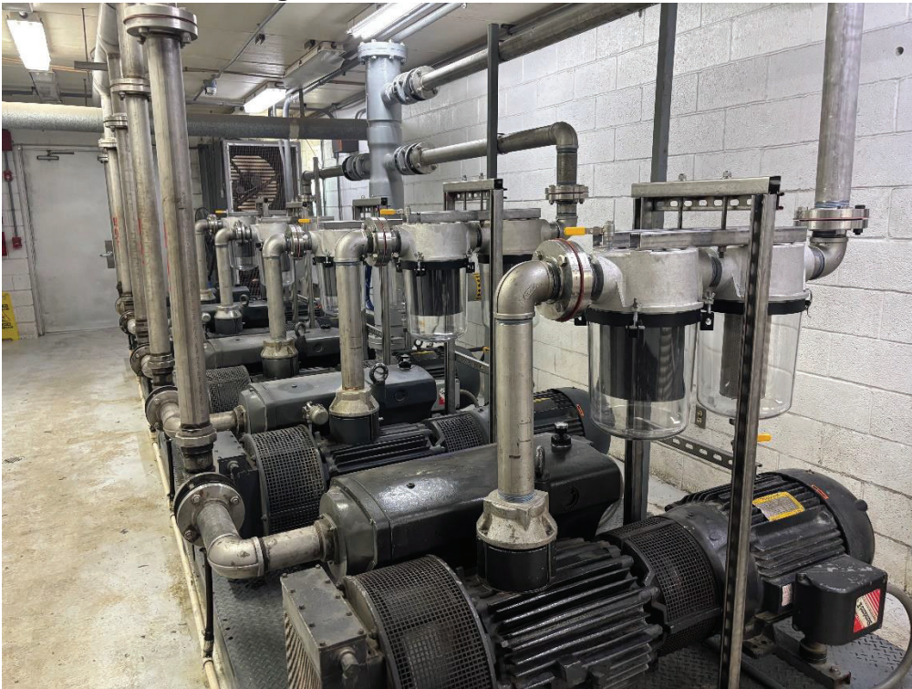
Figure 2: Vacuum station E with all new pump filters and support brackets installed
