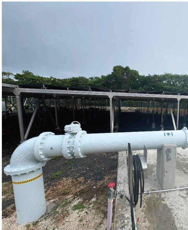
Figures 7 and 8: Well piping treated and painted.
