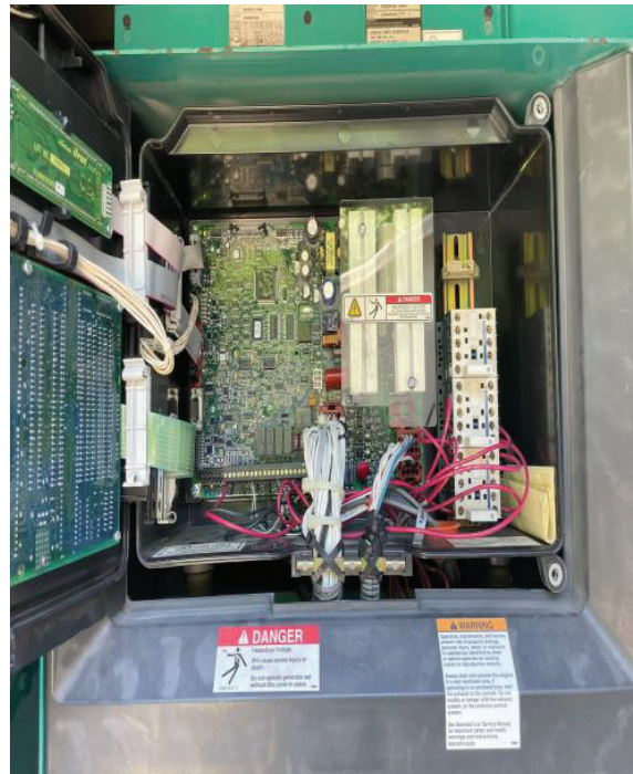
Figures 9 and 10: Vacuum station I backup generator ECU repair
