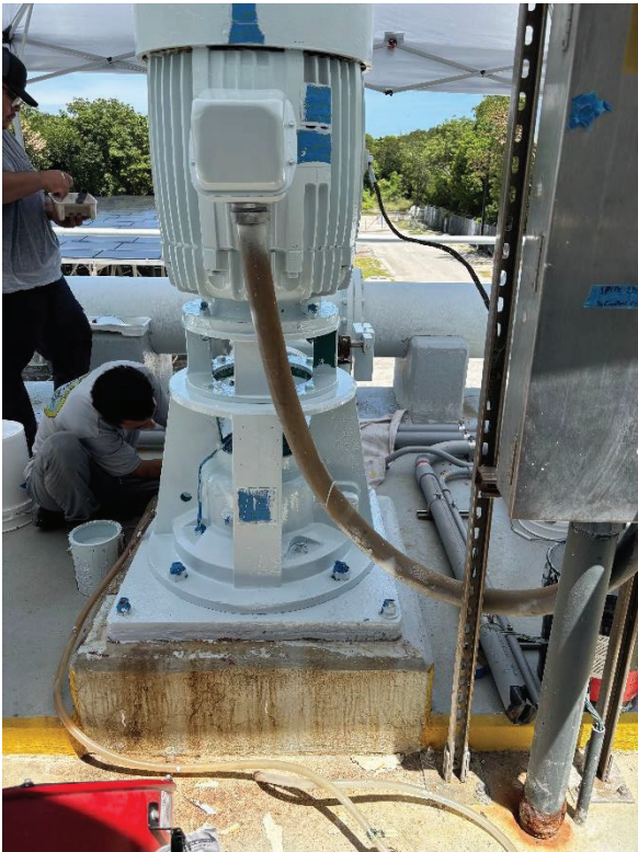
Figures 5 and 6: Injection well pumps treated and painted.
