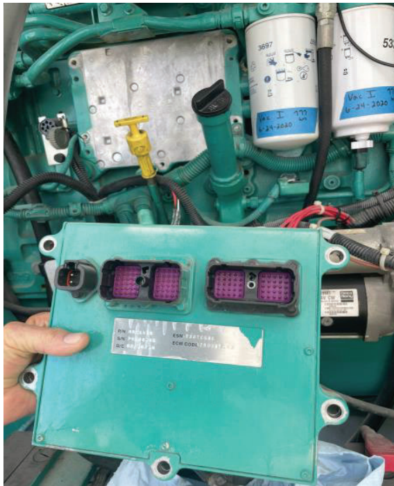
Figures 9 and 10: Vacuum station I backup generator ECU repair
