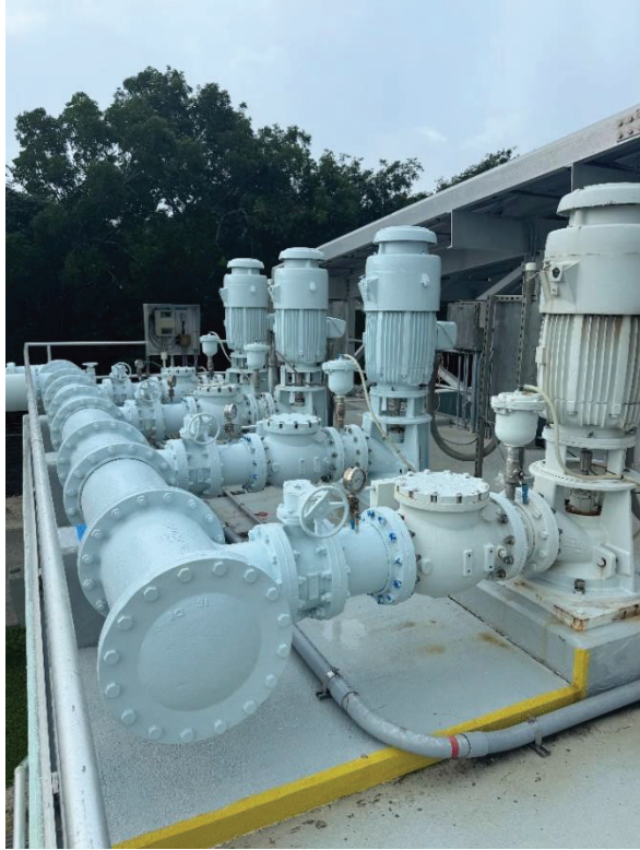
Figures 5 and 6: Injection well pumps treated and painted.
