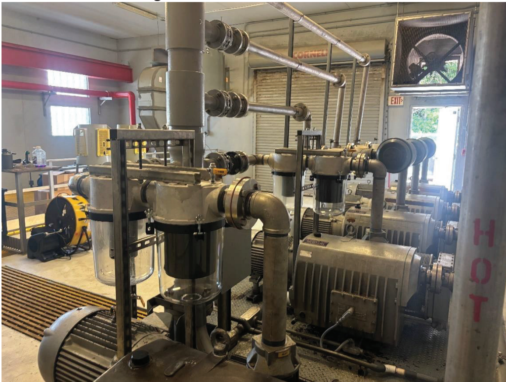
Figure 4: Vacuum station D 2 of 5 pump filters complete
