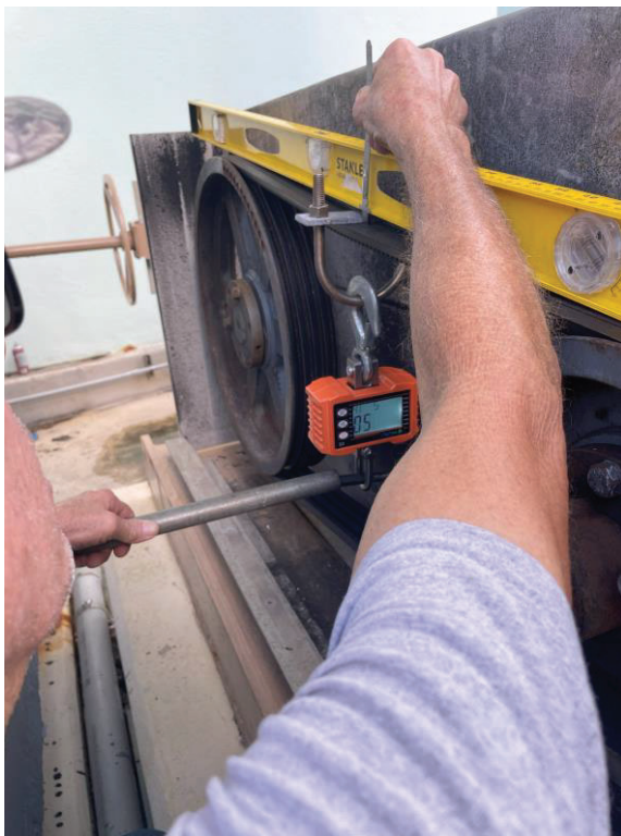
Figure 11: Digester motive pump belt adjustment.
