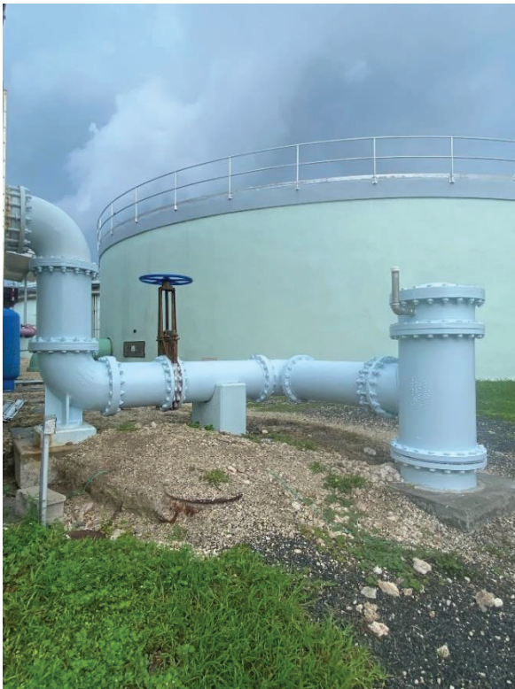
Figures 7 and 8: Well piping treated and painted.
