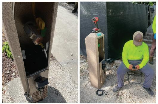
Figures 5 & 6. FloVac Checking Pit is Online After Pulling Hose Lines through Conduit
