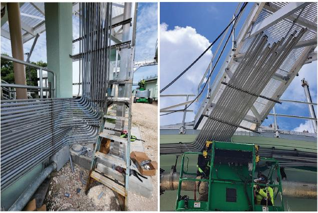
Figure 11 & 12. Conduit Run at Disk Filter Platform & Underneath SBR Tank #3
