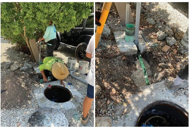
Figures 1 & 2. Collection System Monitoring IVC Concrete Installing Conduit in Trench
