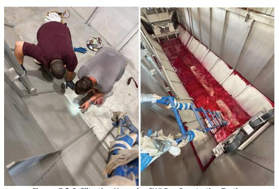
Figures 7 & 8. Filtration Upgrades CWI Dye Penetration Testing
