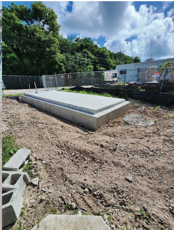
Figures 6 & 7. New Odor Control and Generator Slabs at Vacuum Stations D
