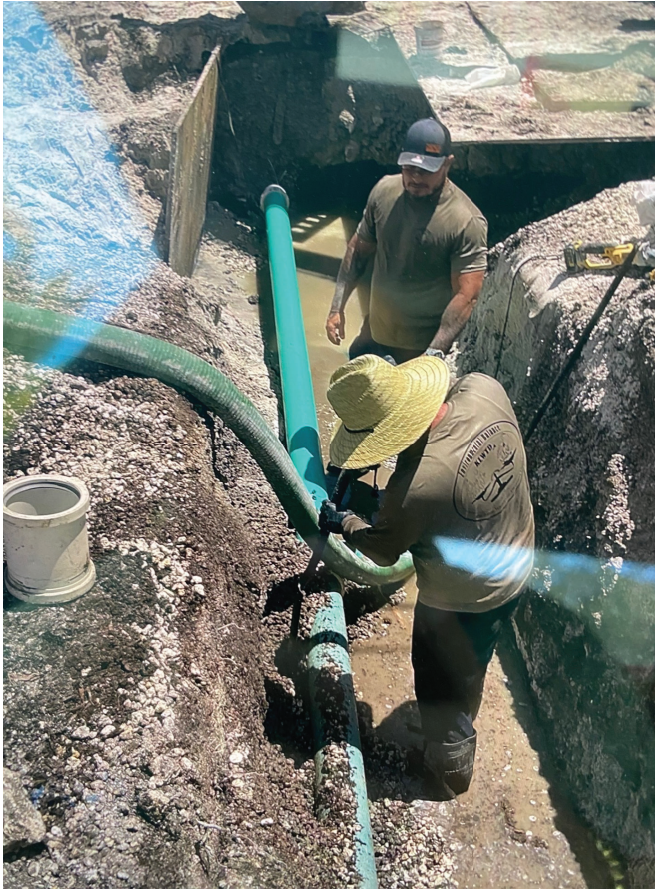
Field Techs assisting contractors at 1000 Shaw Dr. on off setting the lateral service to provide clearance to the Twin Lake drainage project.
