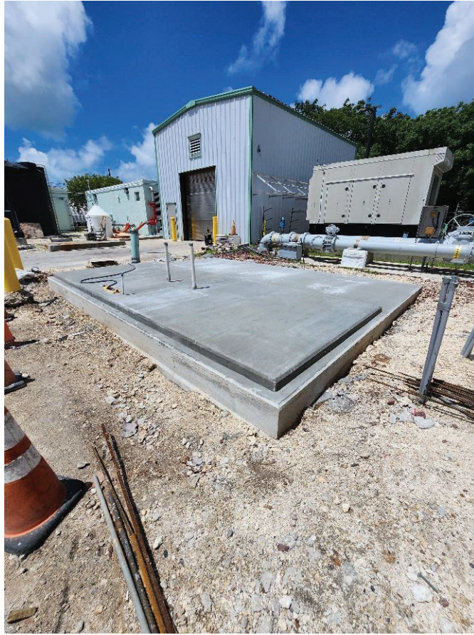
Figures 8. New Odor Control Slab at Vacuum Station E
