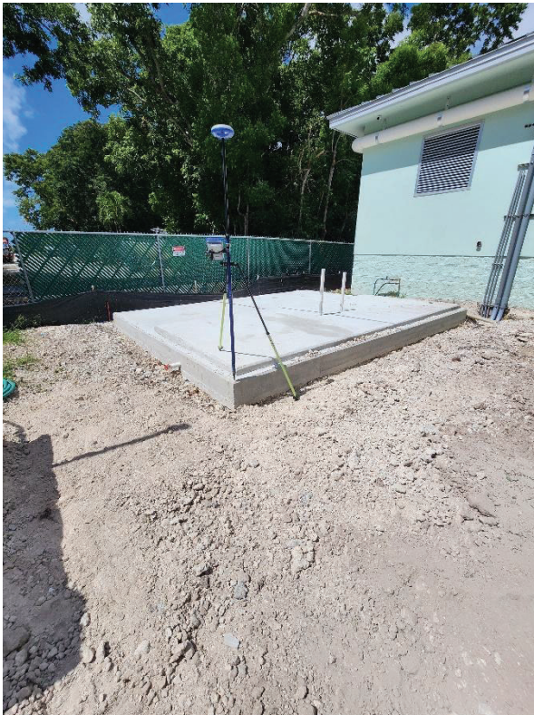
Figures 6 & 7. New Odor Control and Generator Slabs at Vacuum Stations D
