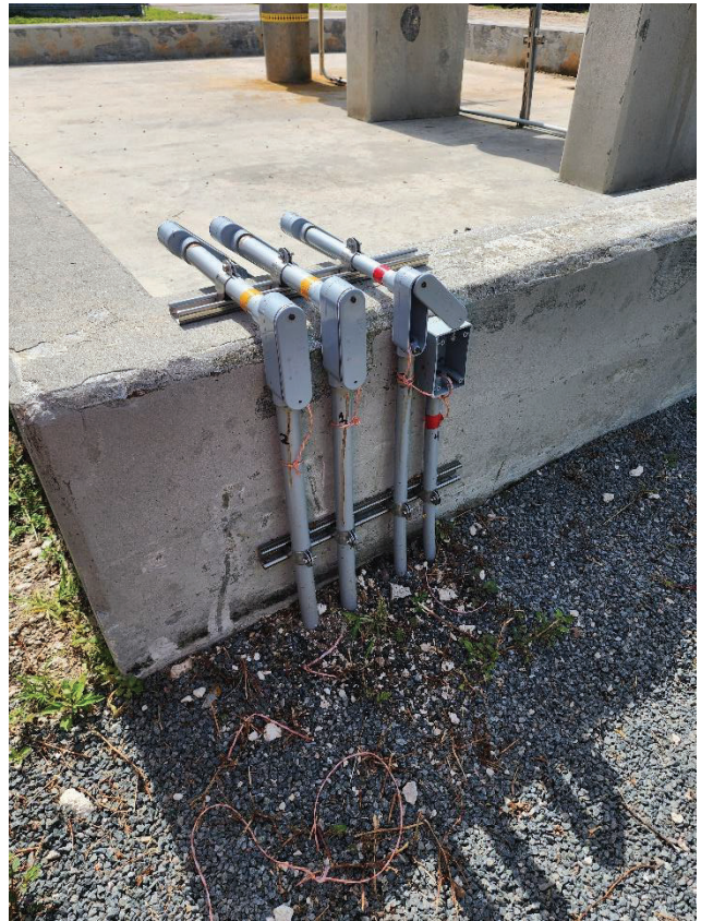
Figure 4 & 5. Barrier Rubber Tape & Wire Pull Strings Installed
