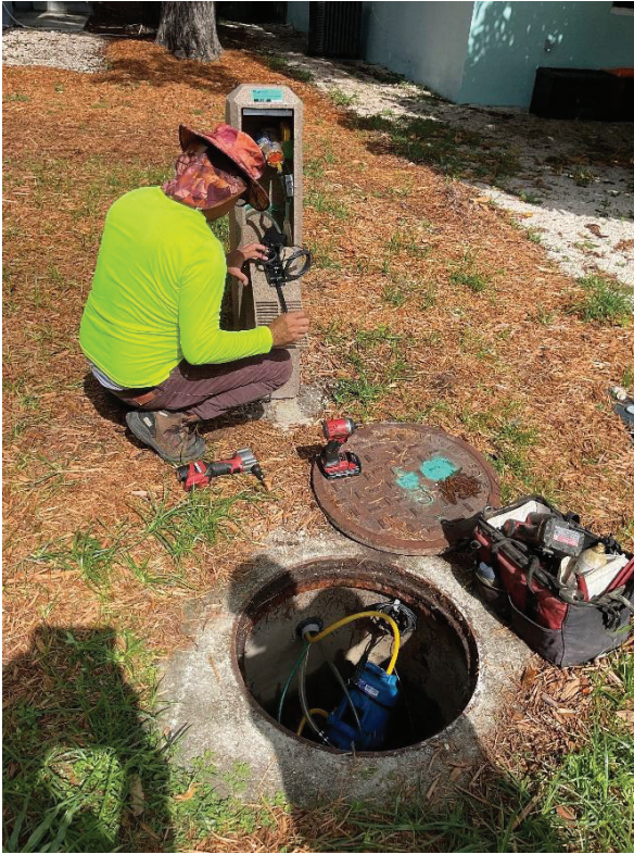
Figures 1 & 2. FloVac Crew Securing Module to Pedestal and Controller and Module Close-up.
