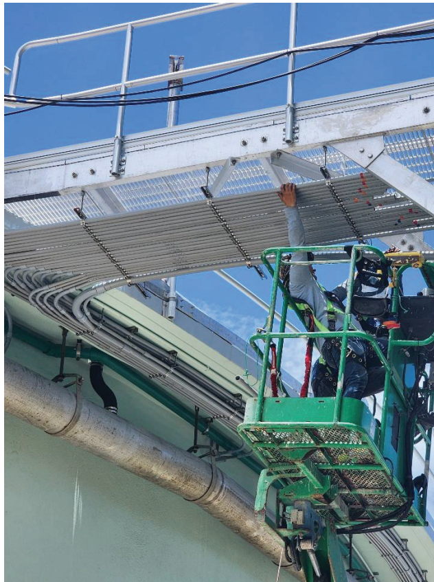
Figure 3. Strapping Conduits to Newly Installed Unistrut Racks Underneath Grate Bridge at SBR #3.
