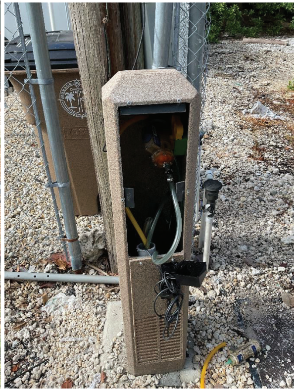
Figures 1 & 2. FloVac Crew Securing Module to Pedestal and Controller and Module Close-up.
