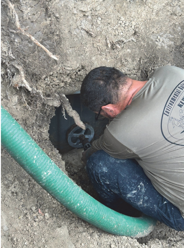
Field Techs tapping into an existing pit to run a new service lateral to 46 Seagate Blvd.
