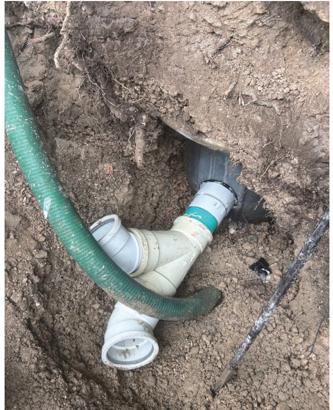
Field Techs tapping into an existing pit to run a new service lateral to 46 Seagate Blvd.
