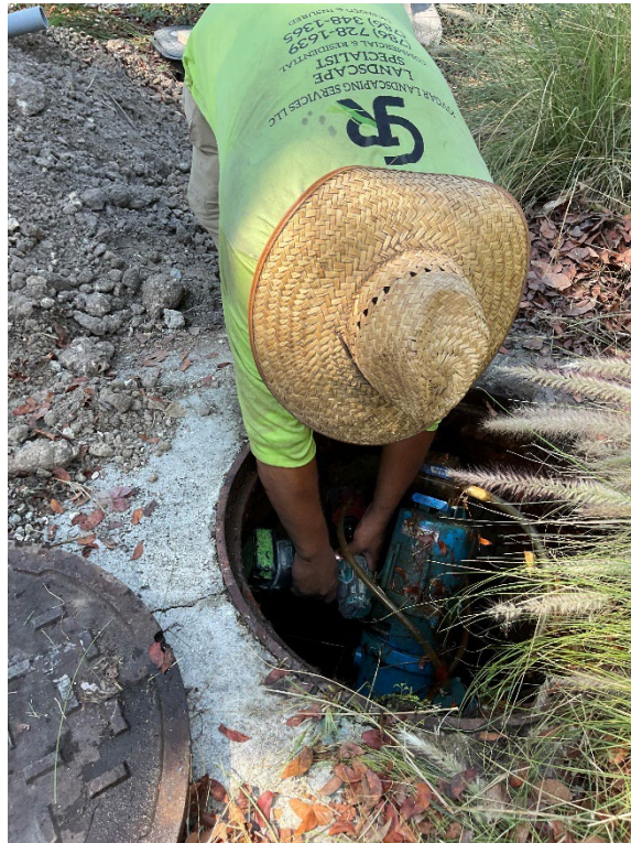
Figure 1. IVC Cutting Hole for Grommet in Sidewall of Pit (318 Belmont Ln.).
