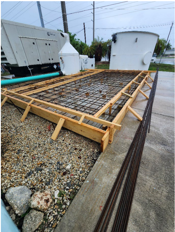
Figure 17 and 18. Rebar and Formwork for the Odor Control Slabs at Station G & I.
