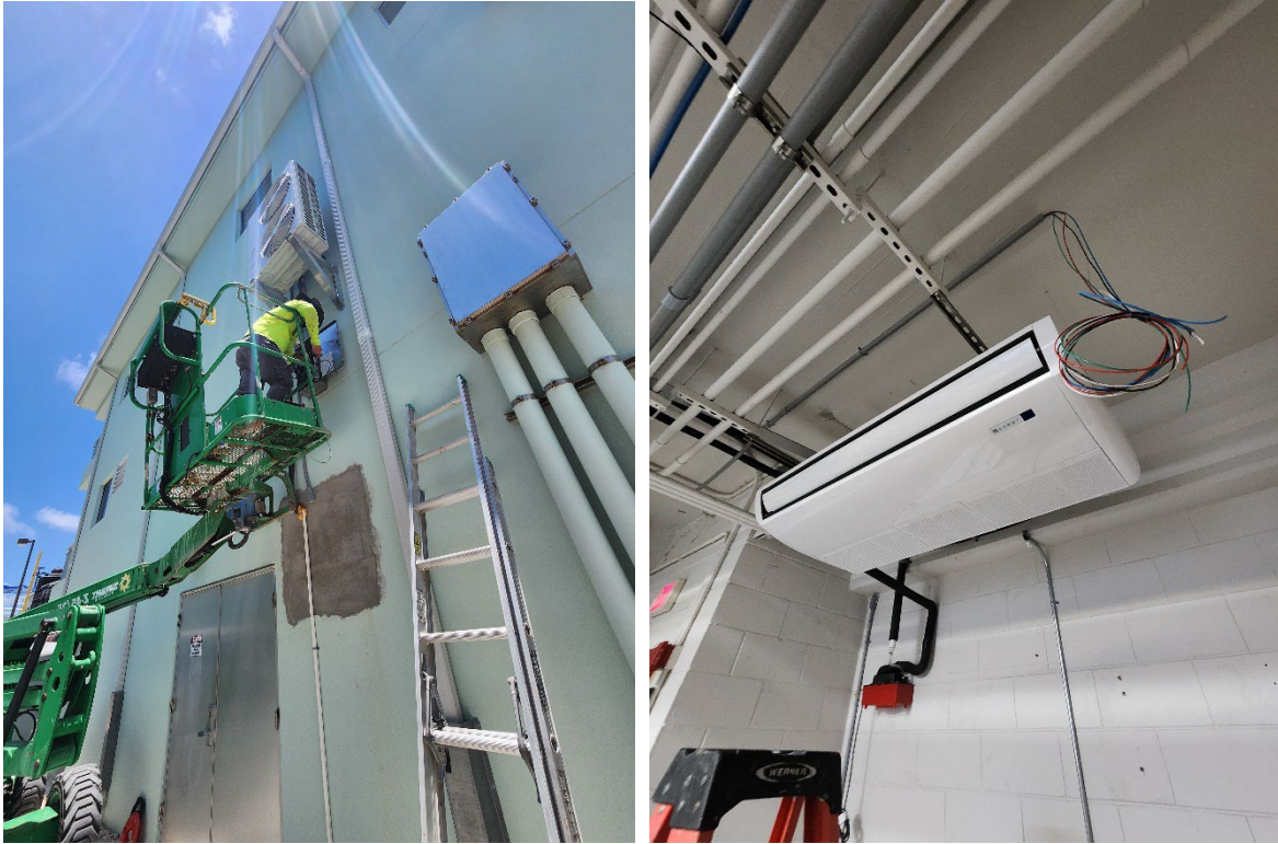
Figure 12 and 13. Running conduit and wires to complete installation of the Mini Split unit.
