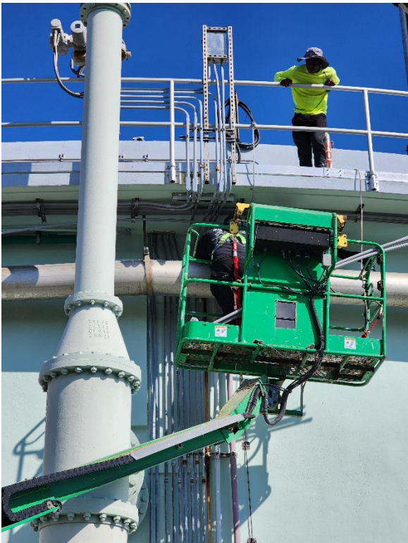
Figure 10 and 11. Conduit stubbed up to both SBRs 2 & 3.
