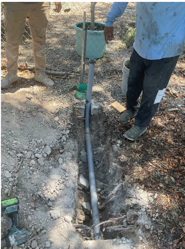
Figure 2 and 3. IVC Crew Installed Conduit in the Trench, and the Compacted the Site Afterward (Hialeah In Basin c)
