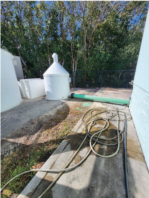
Figure 14 and 15. Odor Control relocation at Vacuum Stations JK and I.
