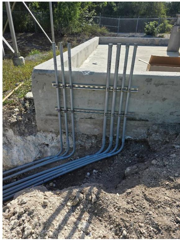
Figure 8 and 9. Conduit stubbed up to both the monitoring and deep injection well
