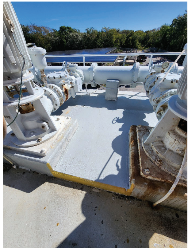
Figure 4 and 5. Newly Coated and Positive Draining Injection Well Pad
