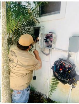
The Low Pressure Monitoring helps provide field staff monitor KLWTD's, Unique Grinder Pump Program. Gives us access to monitor the activations, runtimes and alarms.
