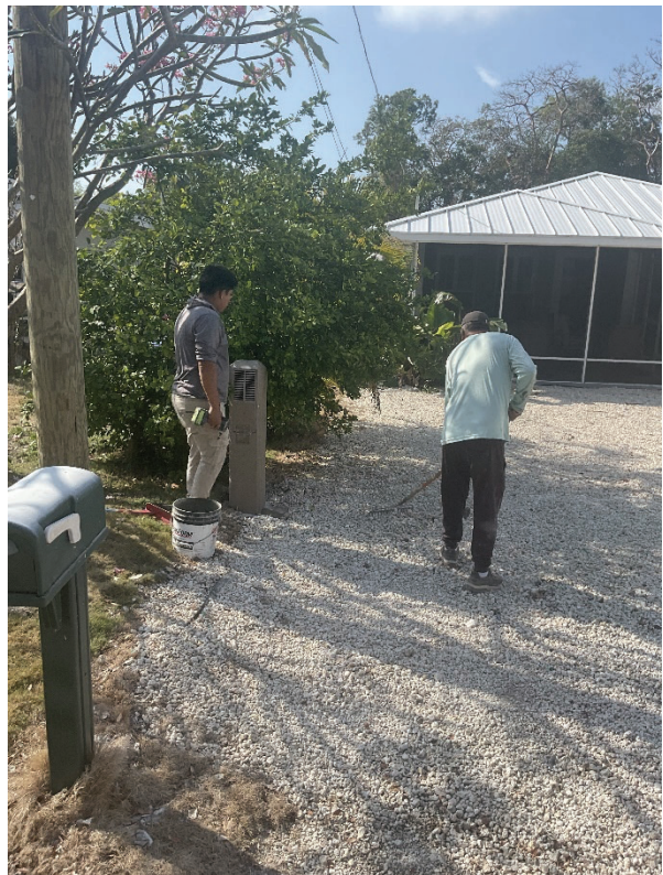
Figure 2 and 3. IVC Crew Installed Detection Tape Over the Conduit in the Trench, and the Compacted the Site Afterward (Plante St. In Basin C)
