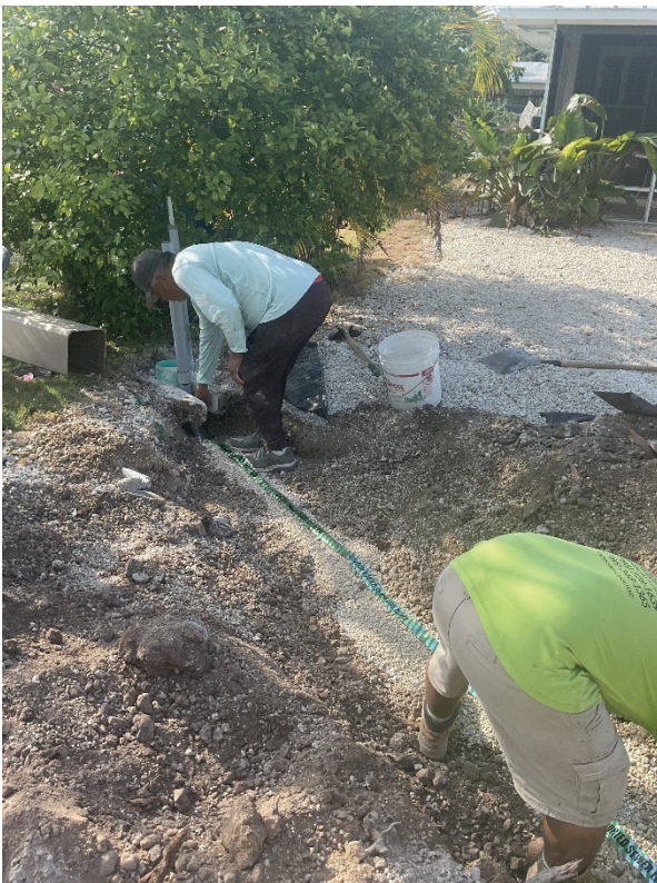
Figure 2 and 3. IVC Crew Installed Detection Tape Over the Conduit in the Trench, and the Compacted the Site Afterward (Plante St. In Basin C)
