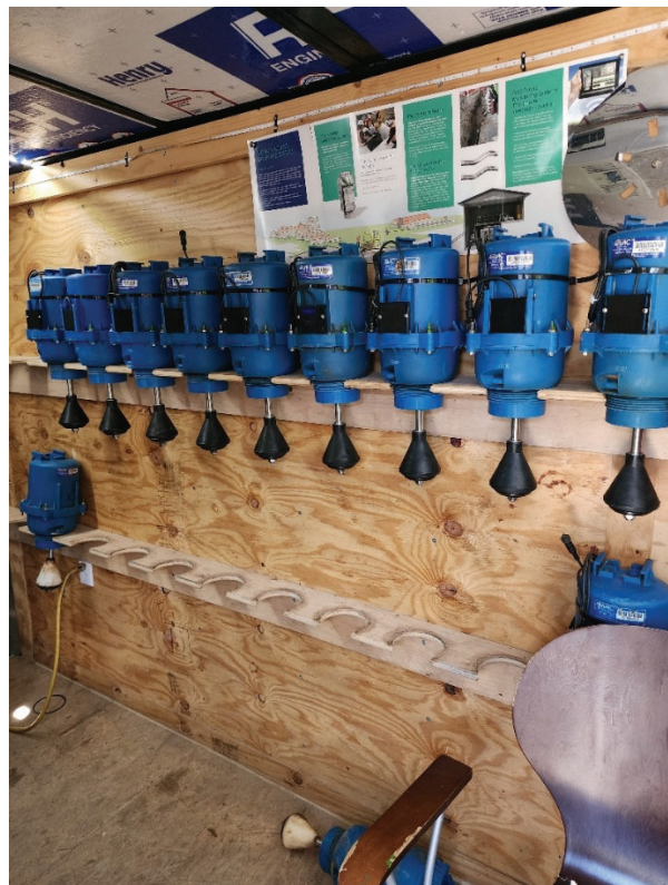
Figure 2. Rebuilt Valve Rack in Flovac Trailer
