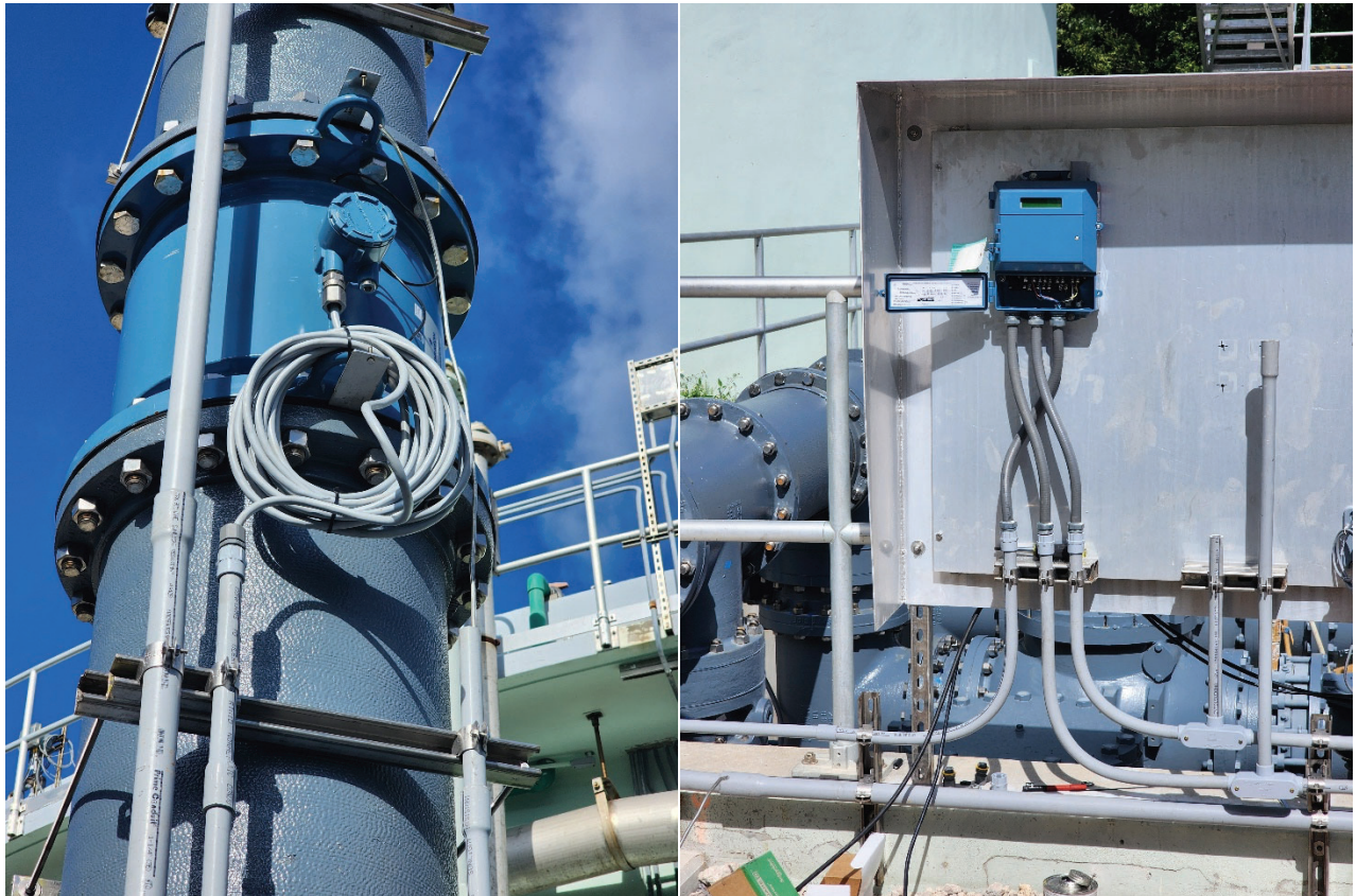
Figure 9 and 10. Conduit Connected to New Flow Meter Display to Flow Meter with Control and Power Wiring
