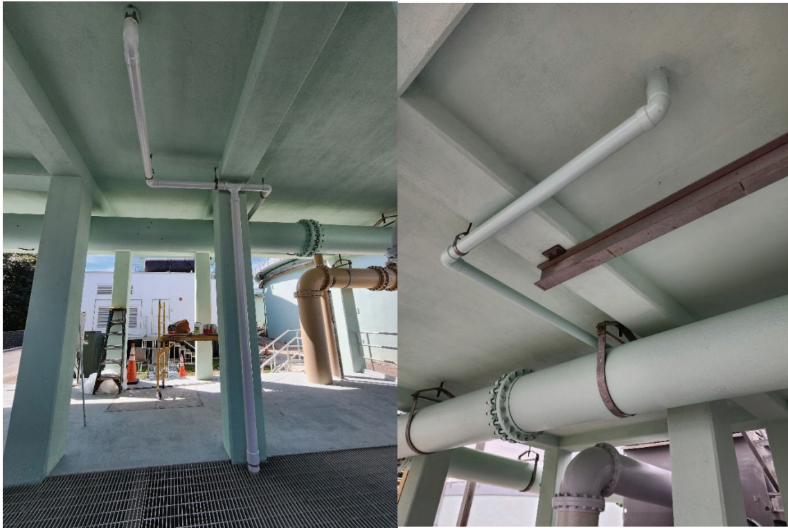
Figure 7 and 8. New Filter Platform Drain Line Installed and Coated
