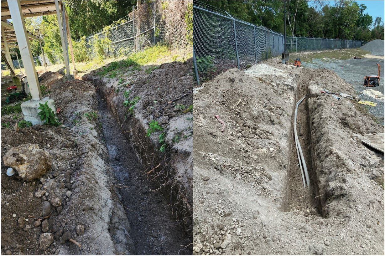
Figure 11 and 12. Exploratory Trenching to Expose Conduits Between Light Poles
