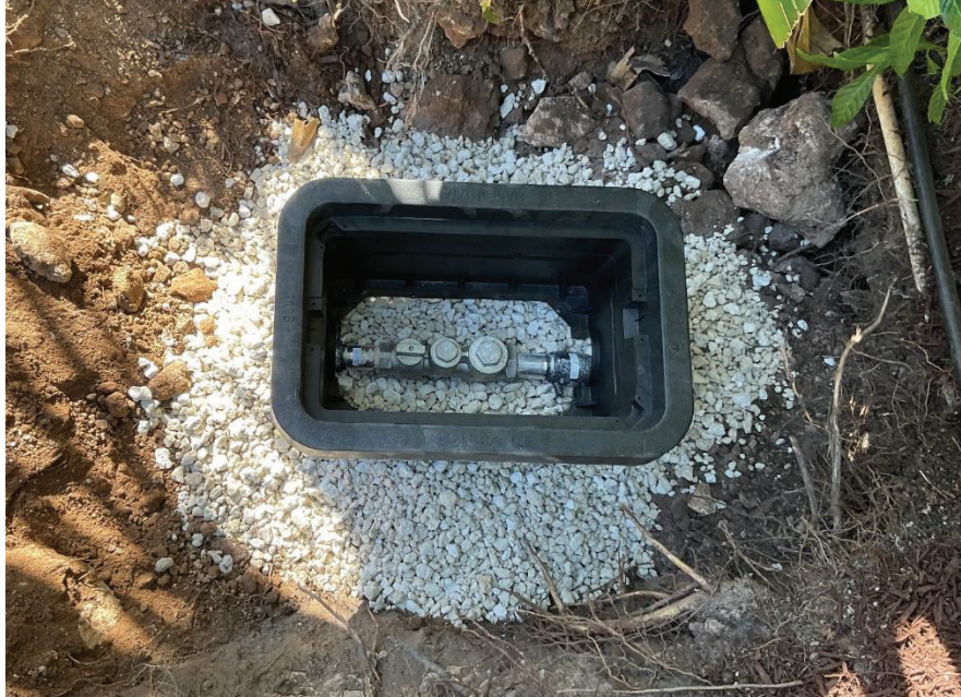
Figure 8. Installation of lateral kits on Coastal Dr.
