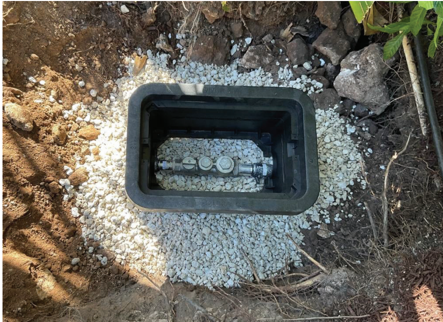
Figure 8. Installation of lateral kits on Coastal Dr.
