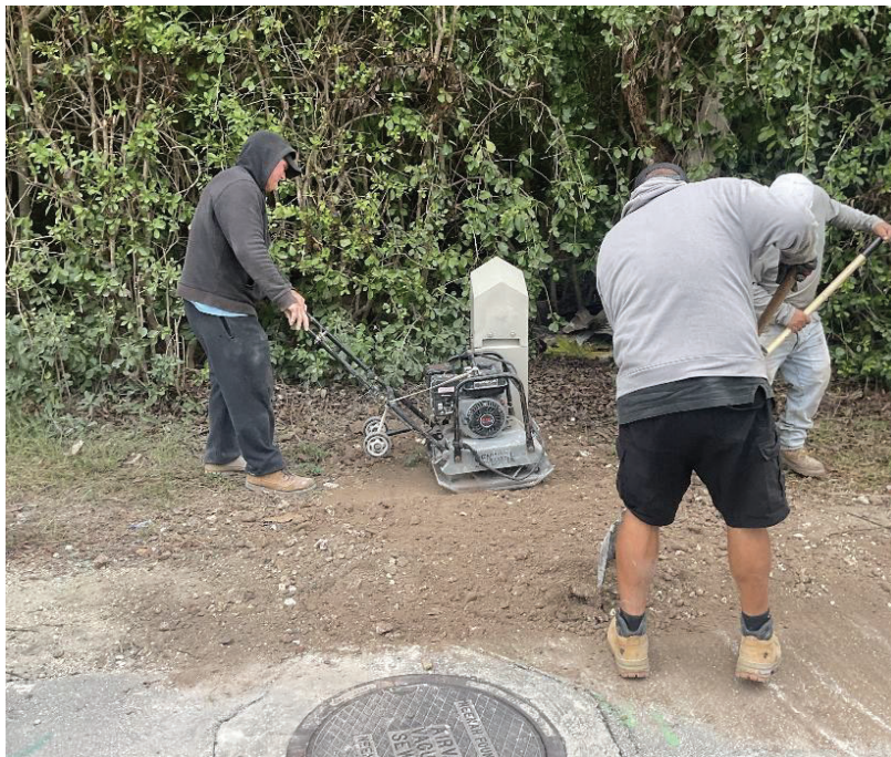
Figure 3. IVC crew compacting the trench with the newly installed conduit, preparing pit for restoration (3/3)
