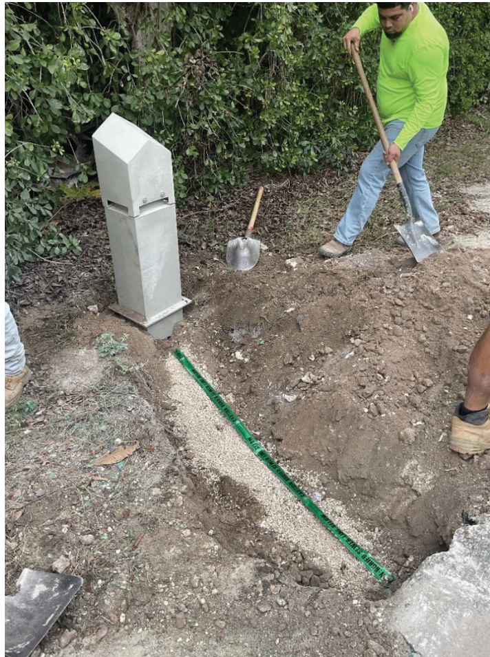
Figure 2. IVC bedding the conduit and installing detection tape (2/3)
