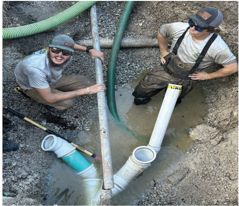
25 Jean LaFitte move clean out and air terminal on to proper right of way
