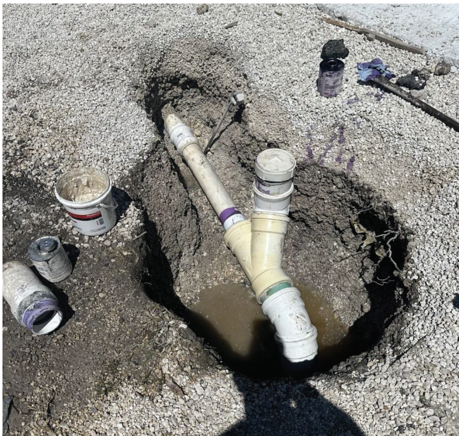
1502 Shaw Dr. Broken clean out repair
