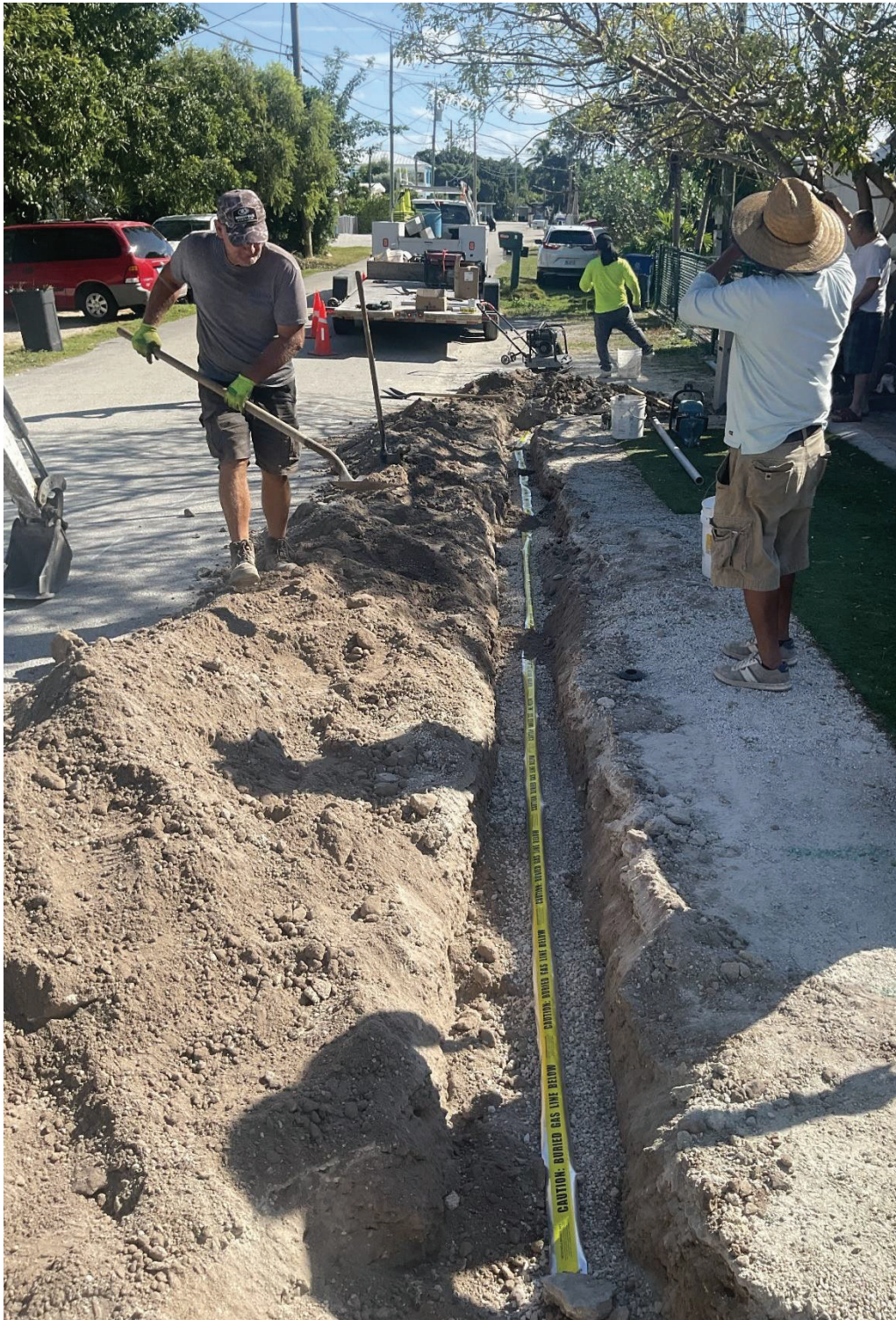
Figure 4. Install Conduit and Detection Tape in Trench for Collection System Monitoring Project.
