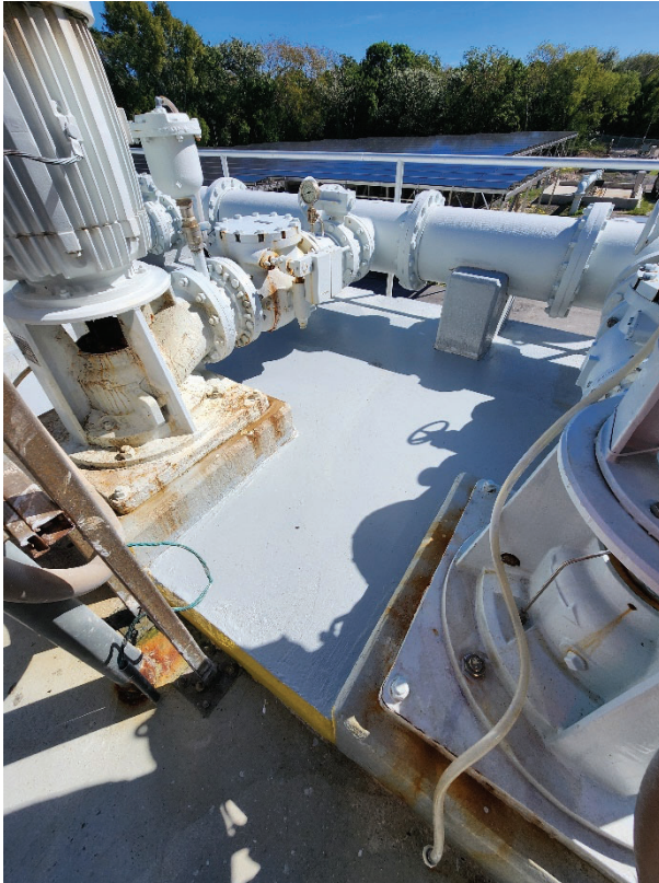
Figure 4 and 5. Newly Coated and Positive Draining Injection Well Pad
