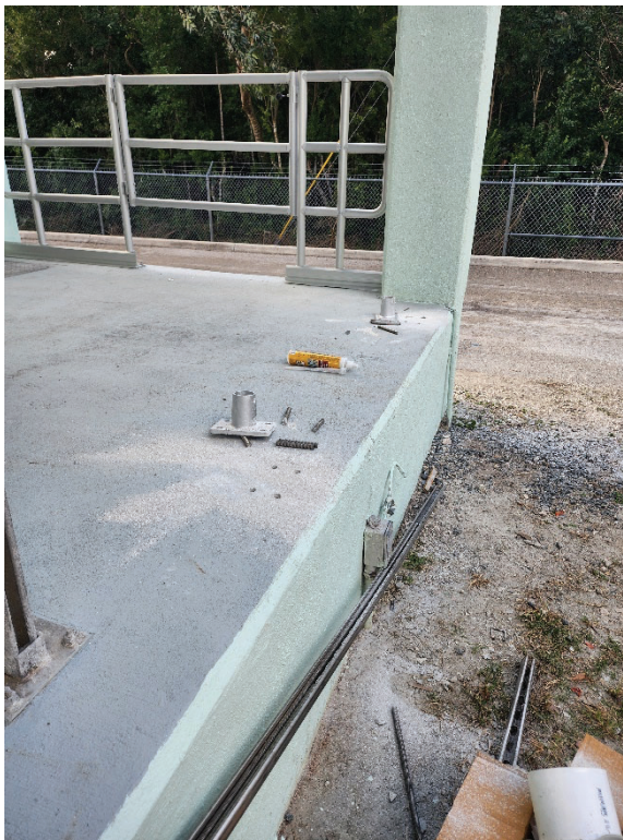
Figure 6 and 7. Placement of New Railings on Bottom of Filter Platform
