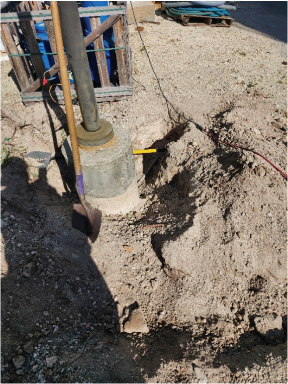
Figure 10 and 11. Exploratory Trenching to Expose Conduits Between Light Poles and Replace with New Conduit and Wires
