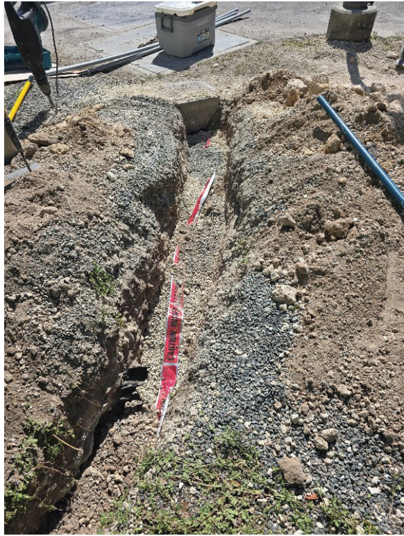
Figure 10 and 11. Exploratory Trenching to Expose Conduits Between Light Poles and Replace with New Conduit and Wires
