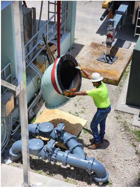
Figure 8 and 9. Crane Removing a Flange to allow for the removal of the 40X Disk Filter.
