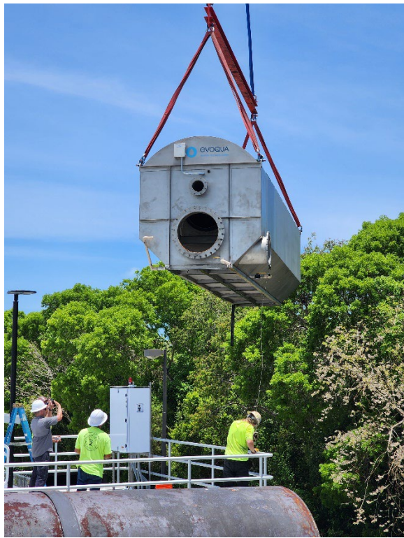
Figure 8 and 9. Crane Removing a Flange to allow for the removal of the 40X Disk Filter.
