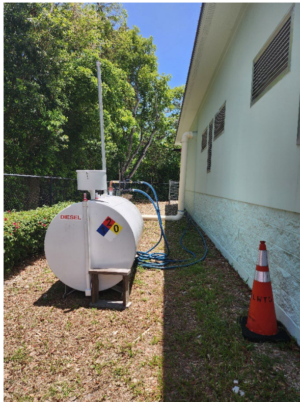
Figure 14. Temporary Fuel Tank has been installed at Vacuum Station A by BOI and passed pressure testing.
