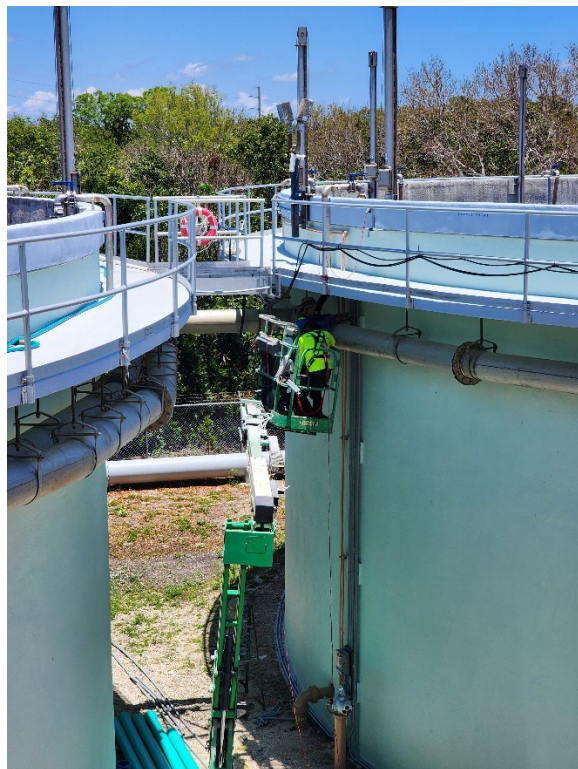
Figure 10 and 11. Conduit stubbed up to both SBRs 2 & 3.
