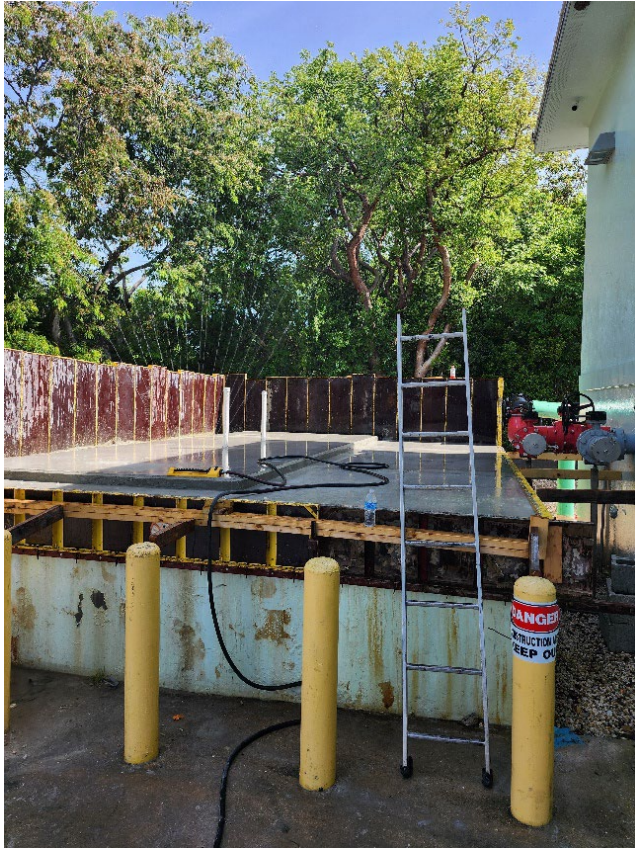
Figure 15 and 16. Odor Control Slab curing at Vacuum Station JK. Coating occurring next period.
