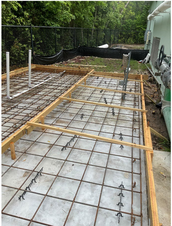
Figure 17 and 18. Rebar and Formwork for the Odor Control Slabs at Station G & I.
