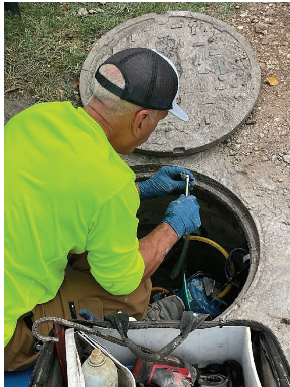
Figure 1. Flovac Crew Installing Vacuum Pit Monitoring Equipment in Basin C (SE Marlin Ave)
