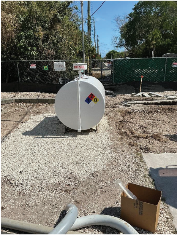
Figure 12 and 13. Temporary Fuel Tank has been installed at Vacuum Station D by BOI and passed pressure testing.
