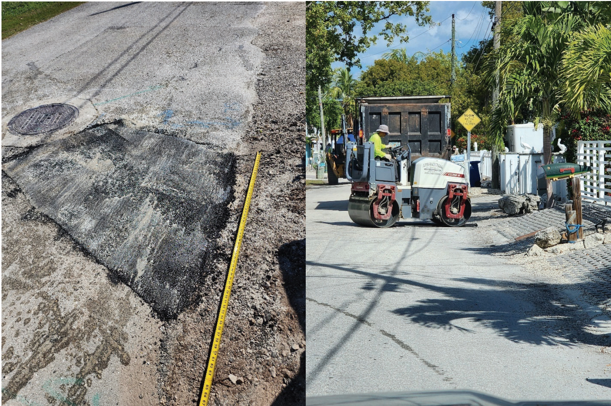
Figure 3 and 4. Compacting Installed Asphalt with Double Steel Wheel Roller/Compactor on #8 Miami Dr.
