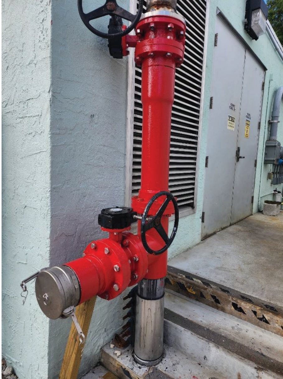
Figure 6. Newly coated odor control piping at Vac E painted in candy apple red from TNEMEC
