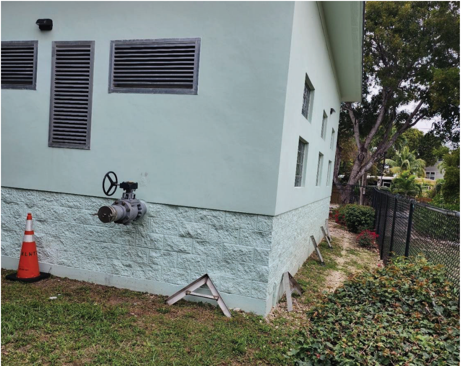
Figure 7. Newly fabricated pipe supports to re-route effluent pipe around to front of building at Vac A
