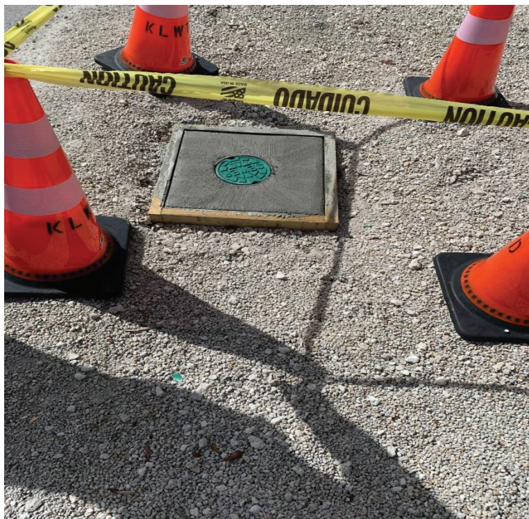
New 6" concrete valve box slab Oakwood and Sexton.
