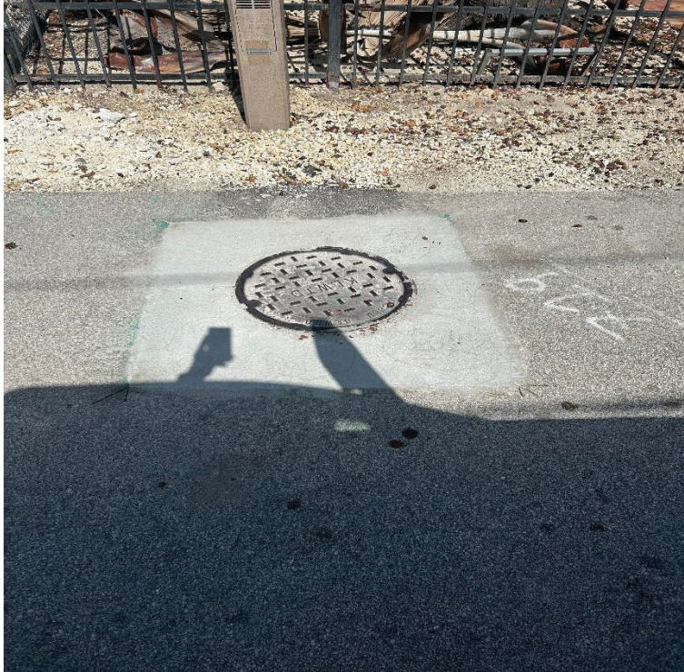
719 Grouper Lane manhole ring damaged and repaired with new ring and 6" concrete slab reinforced with rebar
