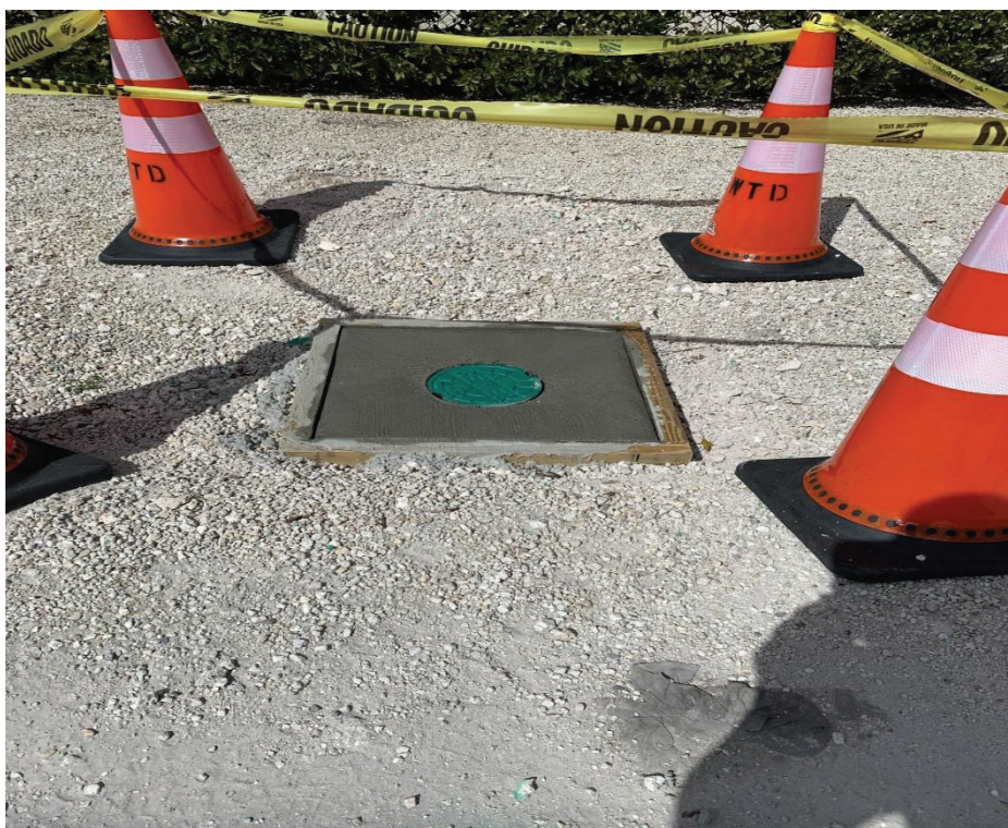
New 6" concrete valve box slab Oakwood and Sexton.
