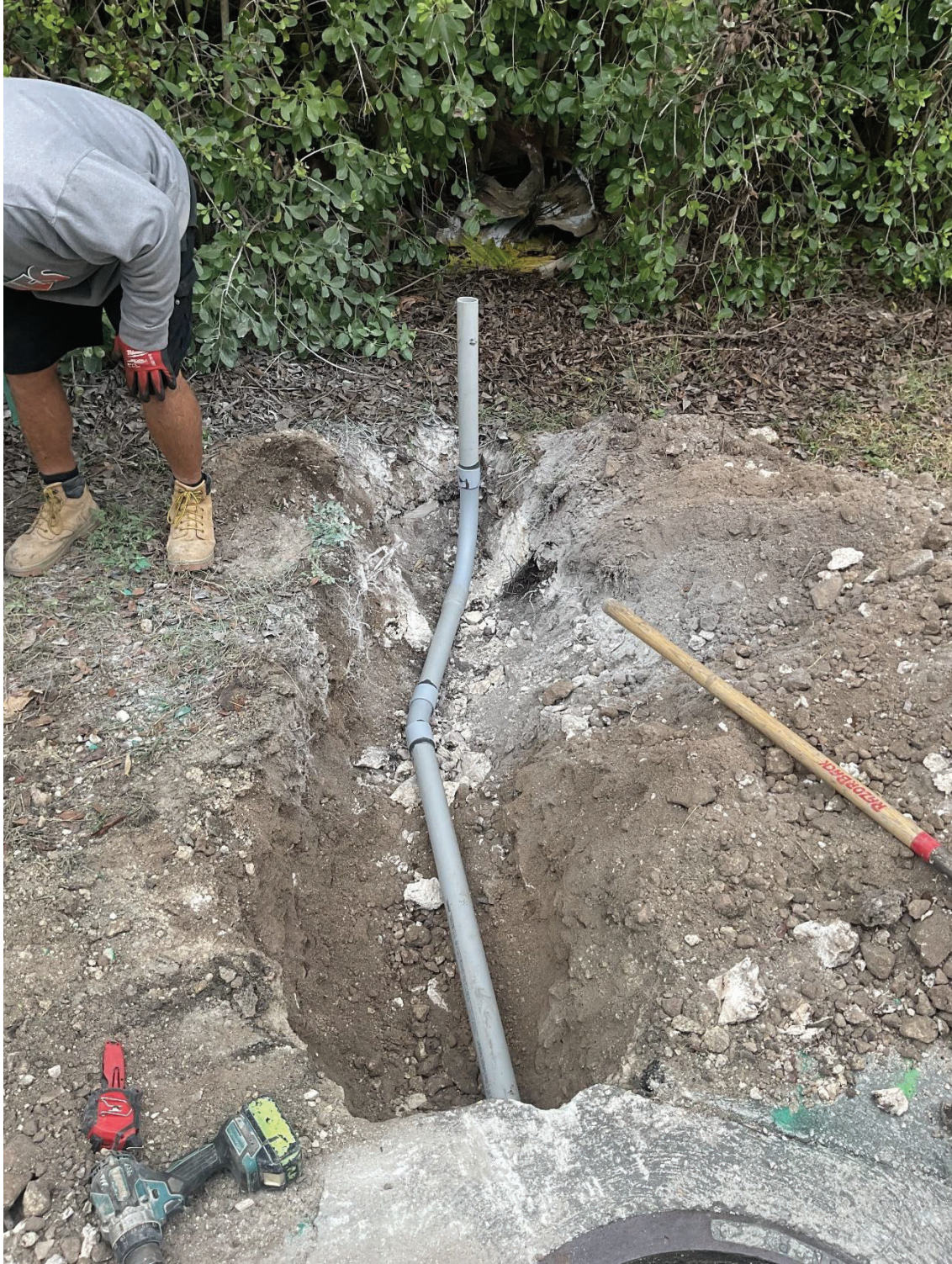
Figure 1. IVC installing conduit in the KLWTD ROW for the Flovac monitoring equipment (1/3)
