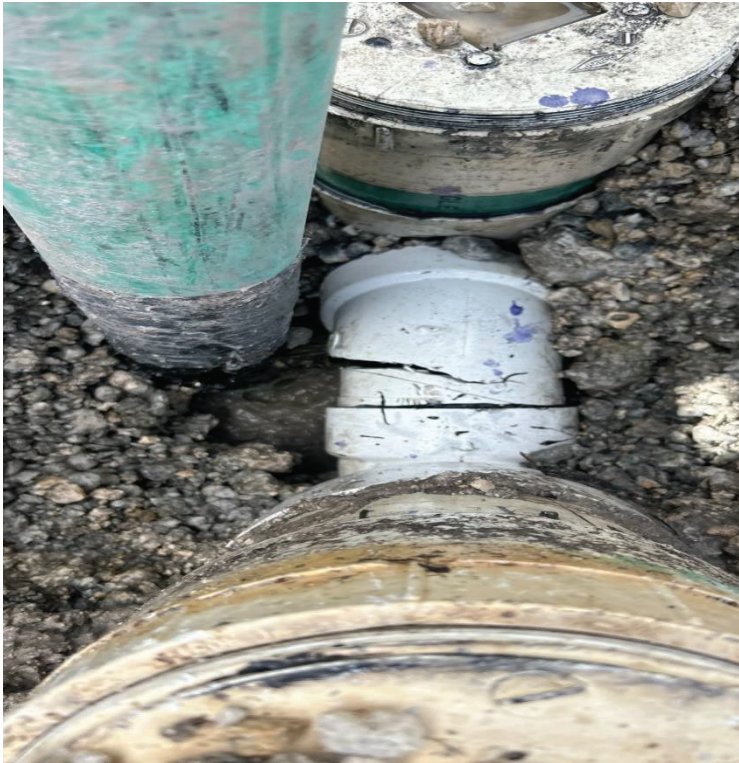
1502 Shaw Dr. Broken clean out repair
