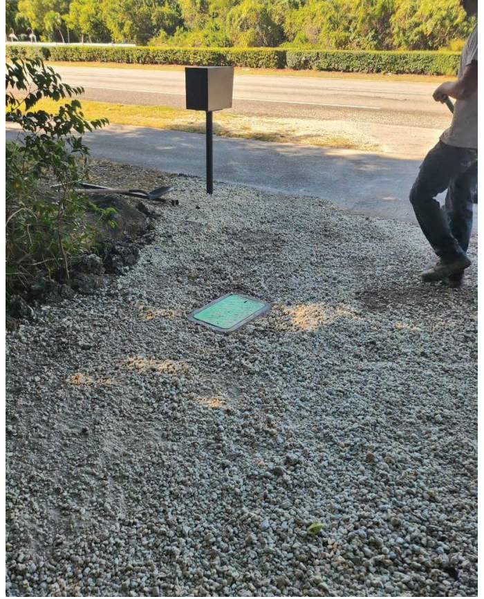
Figure 11. Valve Box Bedded with #57 Stone vs. Fully Installed and Restored
