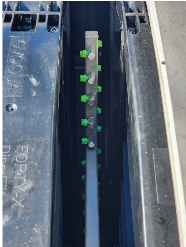
Figure 10. Spray bars and Nozzles Reinstalled Inside Disk Filter Tank
