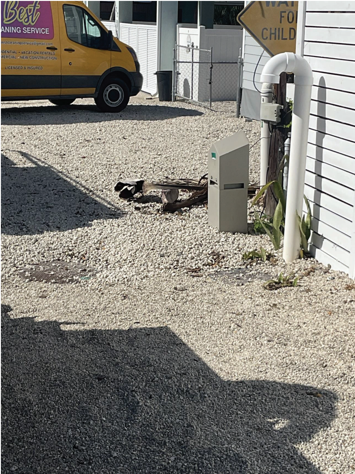
Figure 6. Installed Flovac Pedestal and Candy Cane Dedicated Air Intake – Typical Installation in E0
