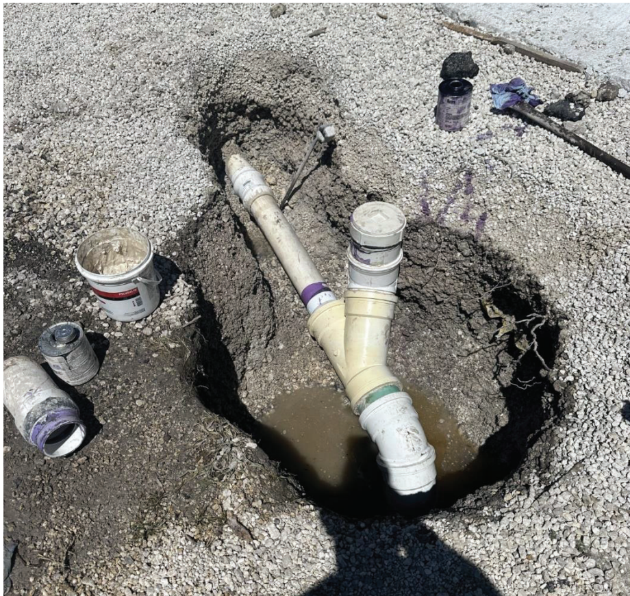
1502 Shaw Dr. Broken clean out repair
