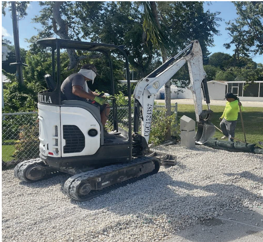
Figure 7 and 8. Installation of Conduit & Flovac Pedestal and Site Restoration for Collection System Monitoring Project
