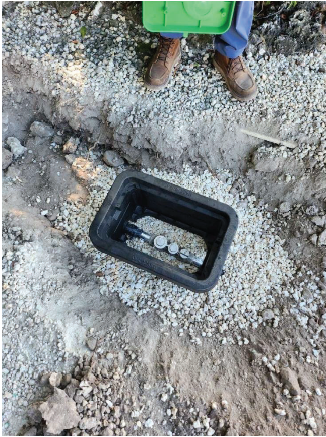
Figure 11. Valve Box Bedded with #57 Stone vs. Fully Installed and Restored
