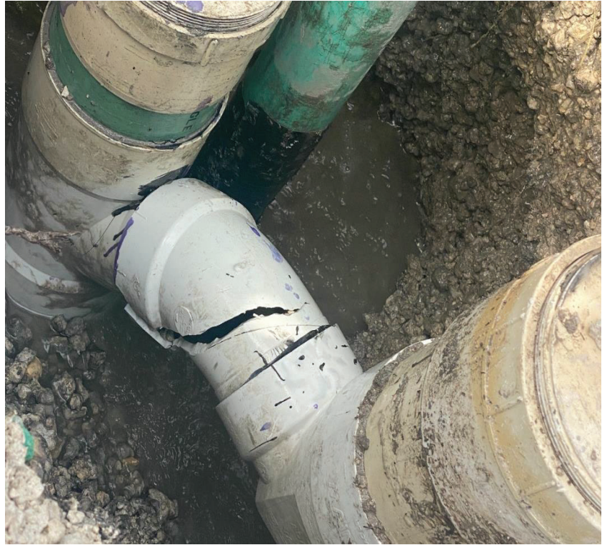
1502 Shaw Dr. Broken clean out repair
