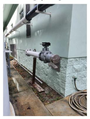
Figure 5. Extended Force Main Connection for Vac Trailer to Corner of Vac G
