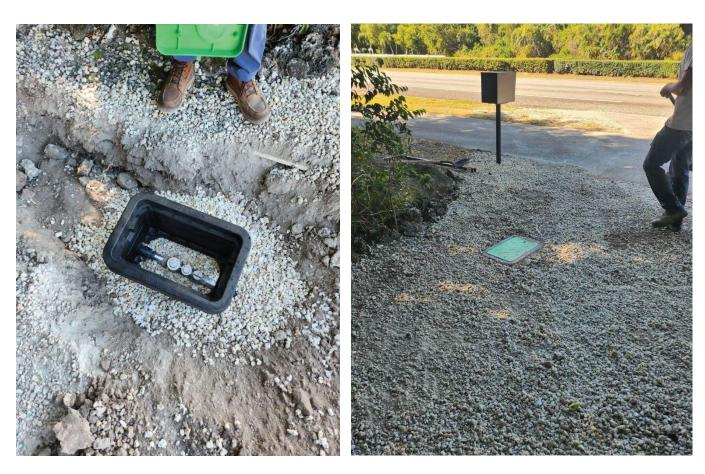
Figure 11. Valve Box Bedded with #57 Stone vs. Fully Installed and Restored
