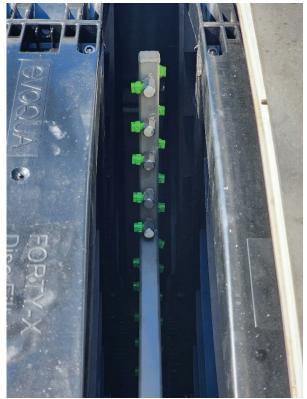
Figure 10. Spray bars and Nozzles Reinstalled Inside Disk Filter Tank
