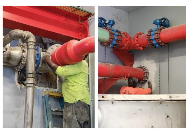
Figure 3 and 4. Patching Pipe-through-Wall Penetrations
